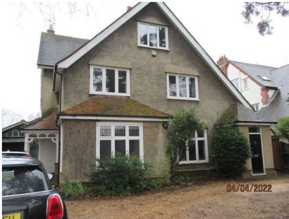
Photo 1 – Main dwelling frontage looking South
