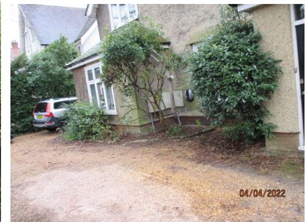
Photo 6 – Frontage looking South east
