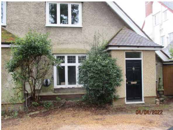
Photo 3 – Existing former porch looking South
