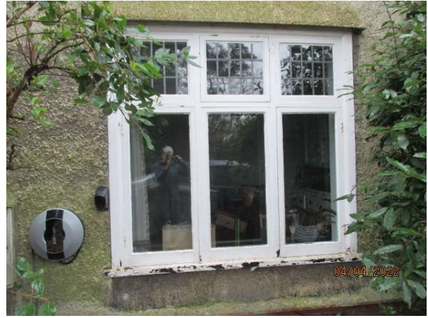
Photo 8 – Existing timber window to Ground floor
