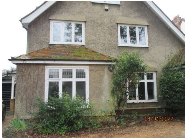
Photo 2 – Frontage of 2 existing windows looking South
