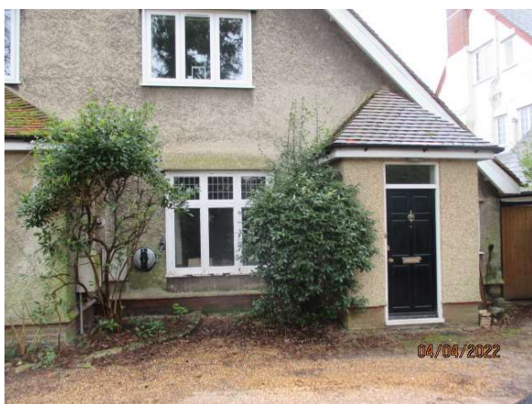
Photo 3 – Existing former porch looking South
