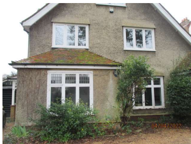
Photo 2 – Frontage of 2 existing windows looking South
