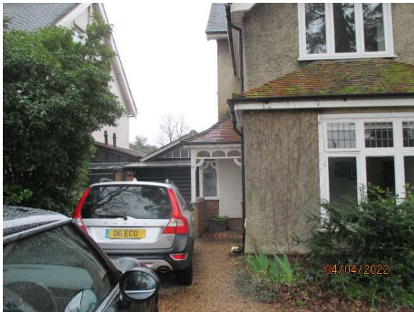
Photo 7 – Existing main side entrance (South)
