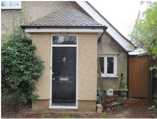
Photo 5 – Existing porch showing door entrance
