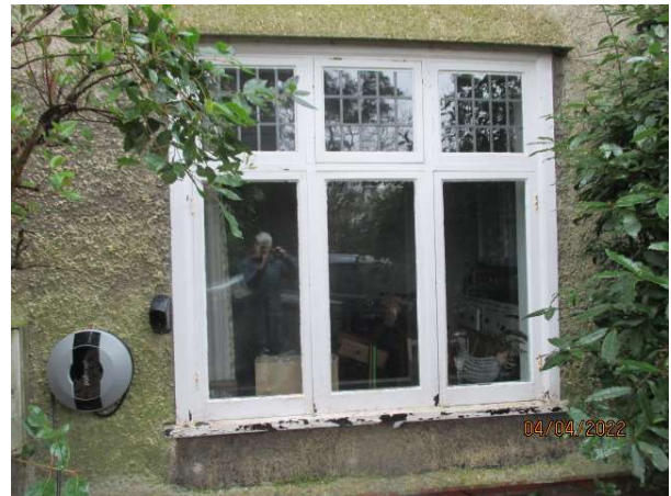
Photo 8 – Existing timber window to Ground floor
