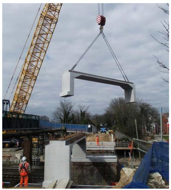
Typical reconstruction of a railway bridge (photograph: C Network Rail)
