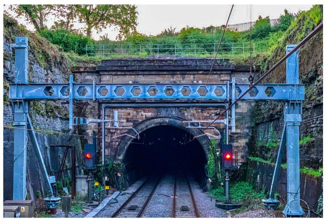
The English portal of the Severn Tunnel (Grade II<sup>\*</sup>), with OLE installed as part of the Great Western Electrification Programme. The OLE support in the foreground was necessary to avoid attaching the OLE to the stonework of the historic portal (photograph: © Furrer+Freyer)
