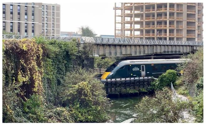
The Intersector Bridge in Cardiff, where new techniques where pioneered to reduce OLE clearances and therefore avoid a very expensive bridge replacement (photograph: © Network Rail)
