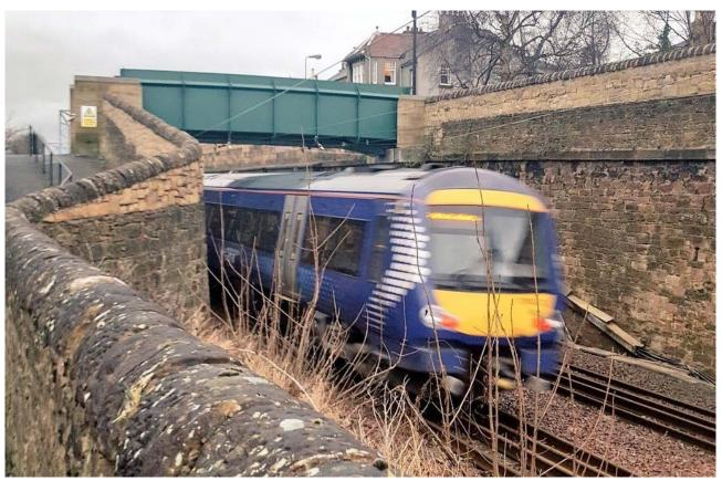
At Linlithgow, boundary walls were sympathetically raised to protect the public from the OLE installed as part of the Edinburgh Glasgow Improvement Programme (EGIP) (photograph: © Network Rail)
