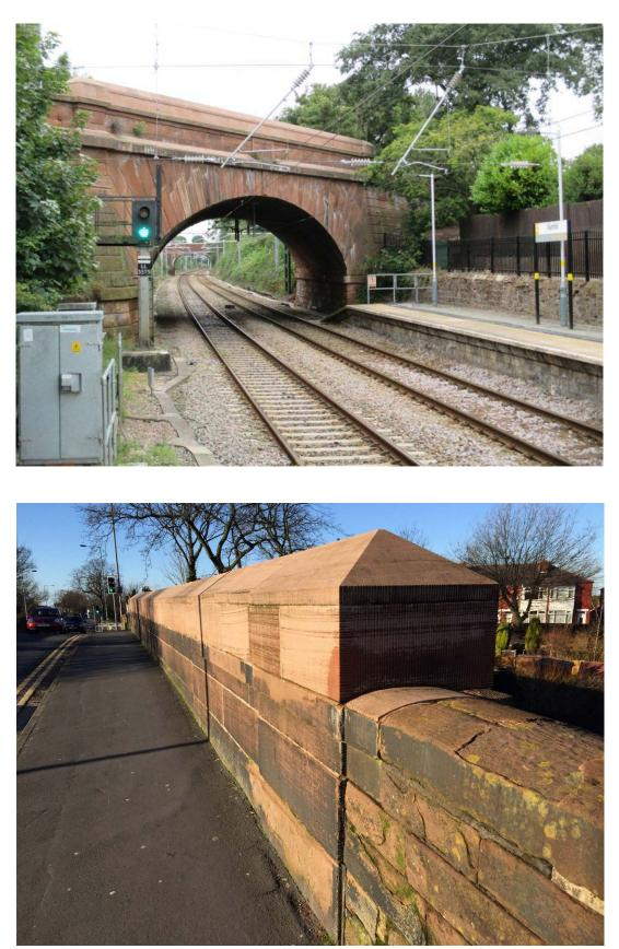
The Rainhill Skew Bridge near Liverpool was designed by George Stephenson as part of the pioneering Liverpool and Manchester Railway in 1830. Recently, the line was electrified and the bridge parapets sympathetically raised. In time, the stone will weather to the same colour (photograph: © Network Rail)
