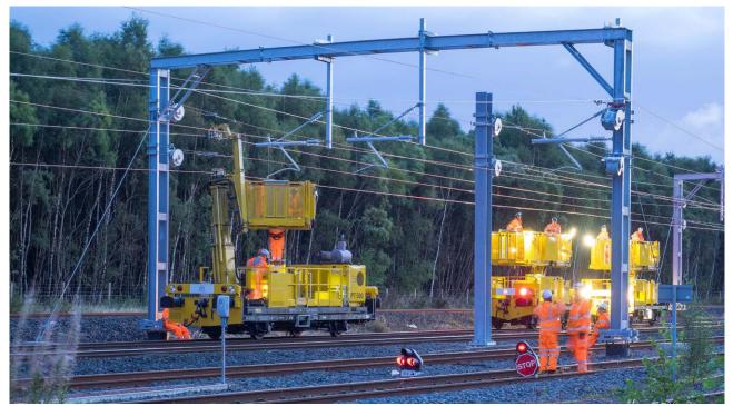
A typical portal frame made of H-section steel members (photograph: ⓒ Network Rail)
