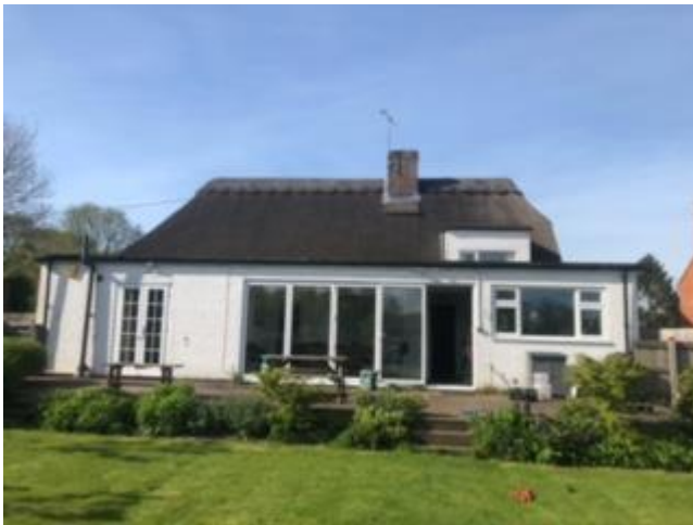
Back view of house & flat roof
