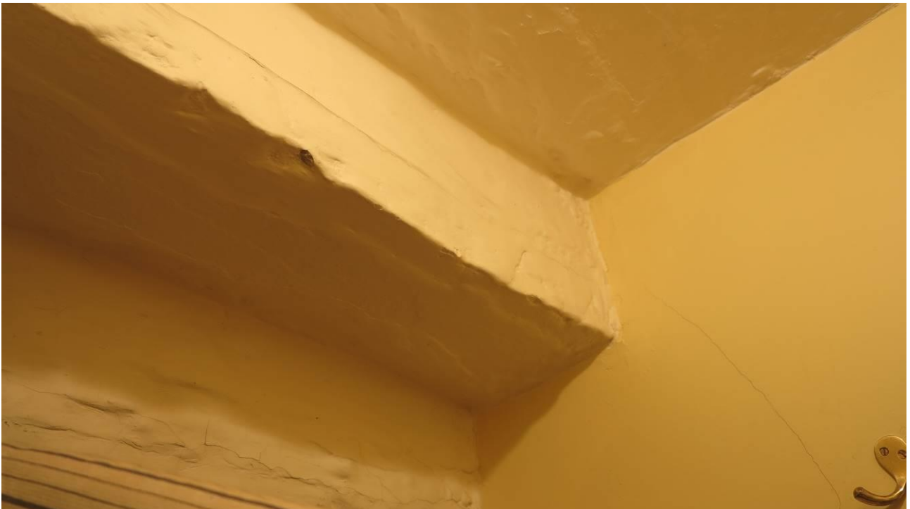
Plate 46. The underside of the staircase is visible in an understairs cupboard
