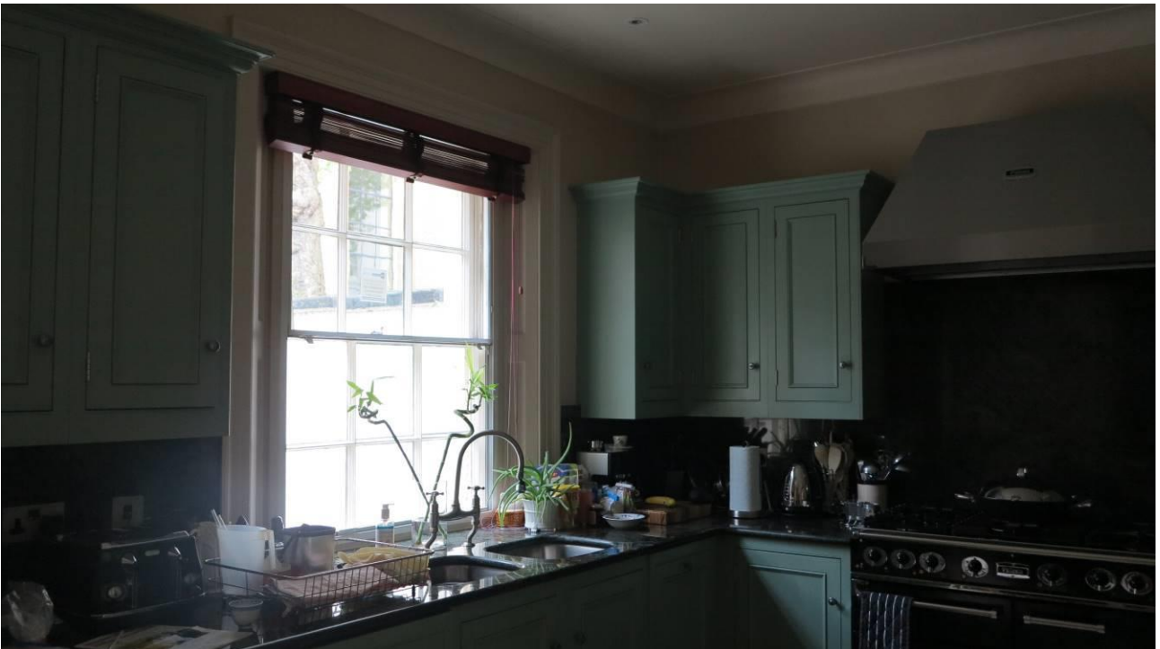
Plate 28. The existing kitchen
