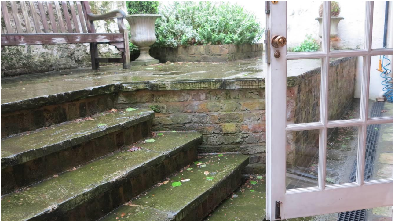
Plate 51. Steps up to rear yard area
