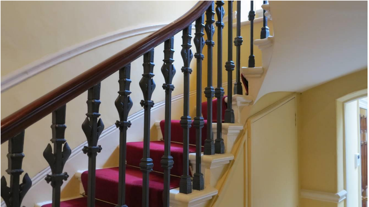
Plate 19. The main staircase, detail of balusters
