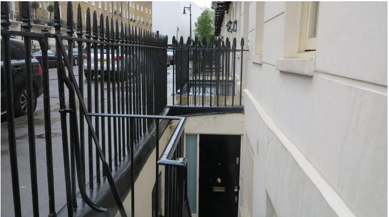
Plate 48. The existing under steps vestibule at No.16 seen from street level
