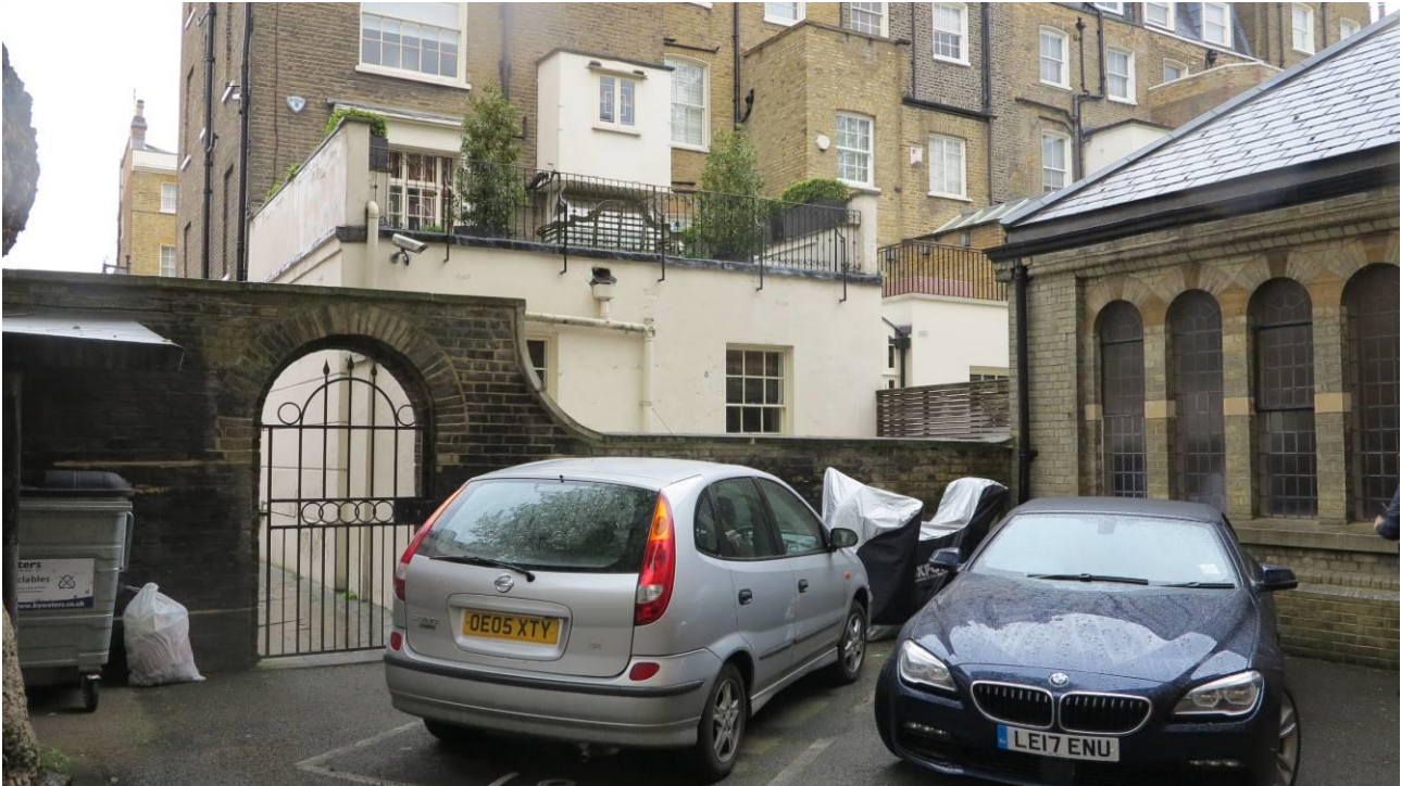
Plate 15. Looking from the grounds of St. Peter's Church, Eaton Square towards the rear elevation of No.16
