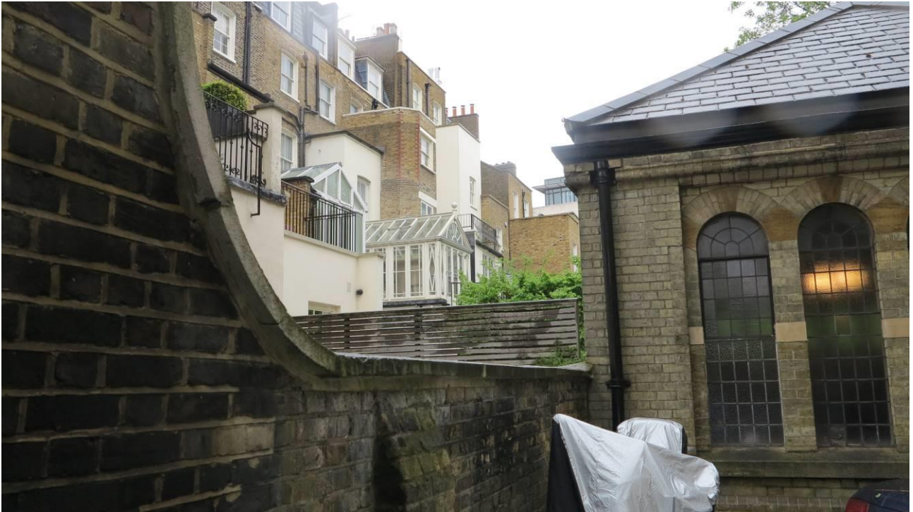
Plate 13. The vestry of St. Peter's Church, Eaton Square backs directly onto the boundary wall separating the grounds of the church from No.16
