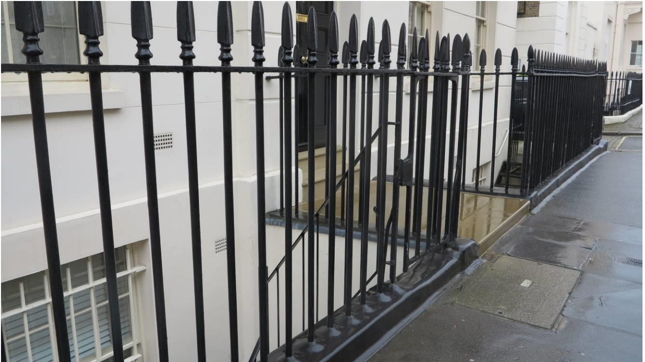
Plate 47. The area to Nos.16 & 17 seen from street level
