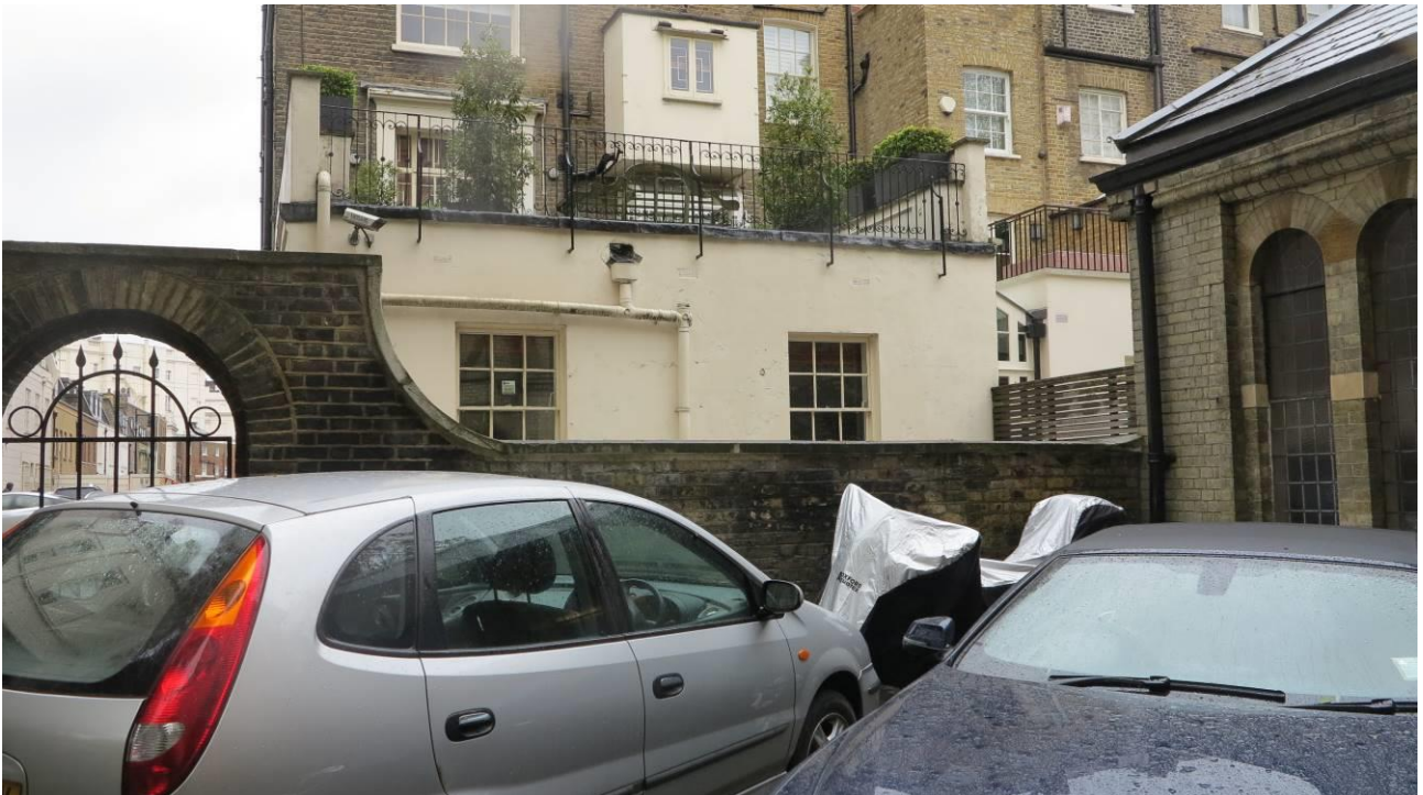
Plate 2. The rear elevation of No.16 seen from the grounds of St. Peter's Church, Eaton Square
