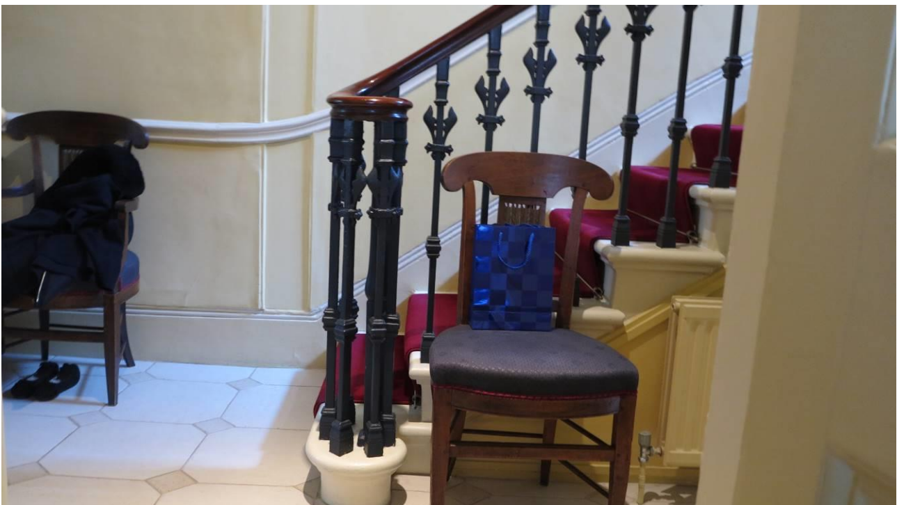
Plate 18. The main staircase, detail of bottom 'newel' and balusters
