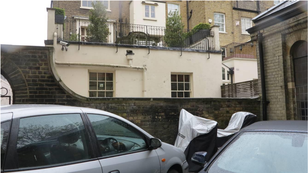
Plate 3. The rear elevation of No.16 seen from the grounds of St. Peter's Church, Eaton Square
