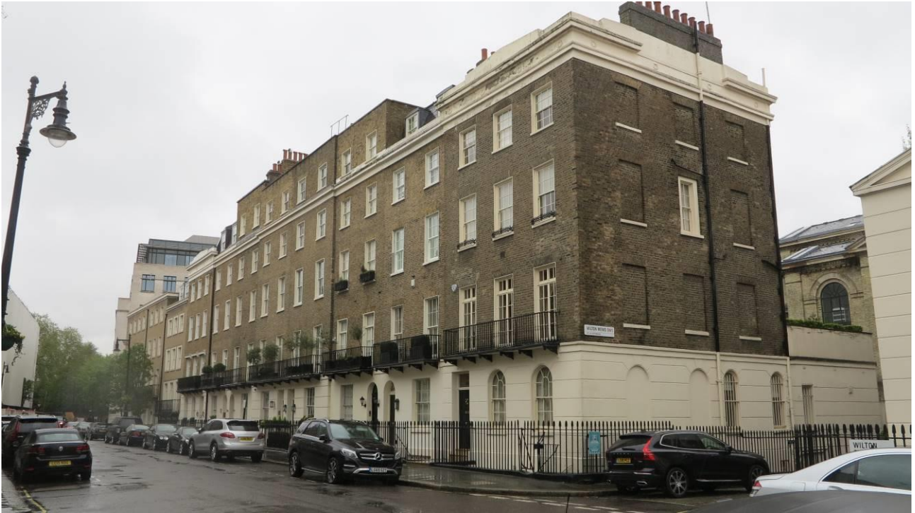
Plate 1. Wilton Street and Wilton Mews elevations of Nos.16-23; No.16 in foreground
