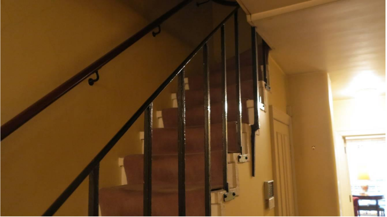
Plate 43. The staircase between the lower ground floor and ground floor
