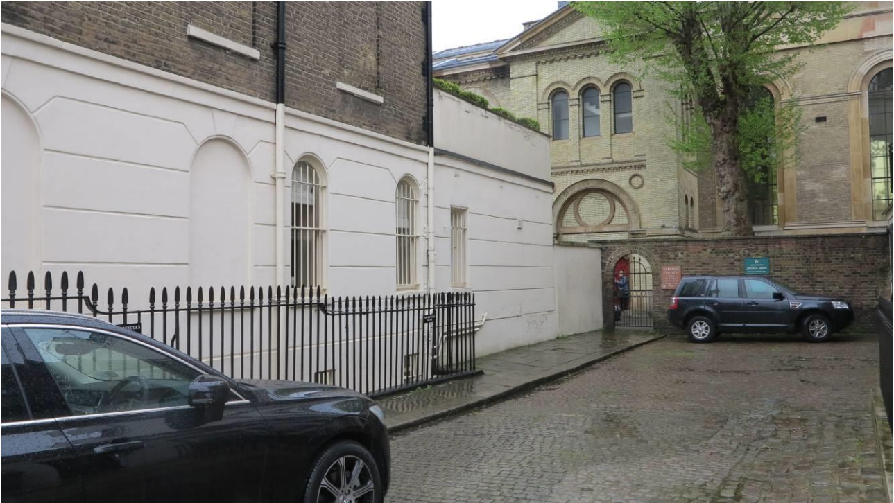
Plate 7. The flank (Wilton Mews) elevation to the rear extension to No.16 and the boundary wall to its rear yard area
