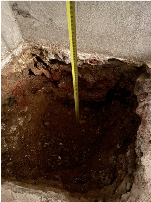
Trial hole to northeast corner of vault below pavement
