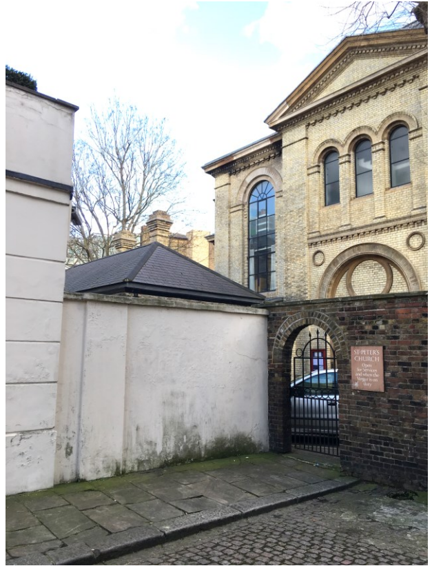
2 View from Wilton Mews of side wall onto lower Courtyard, with St. Peter's Church and vestry beyond
