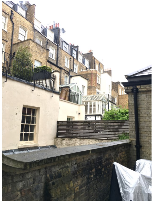
2 View of rear elevation from St. Peter's churchyard
