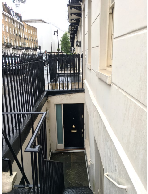
2 View of lightwell fronting Wilton Street showing modern entrance porch
