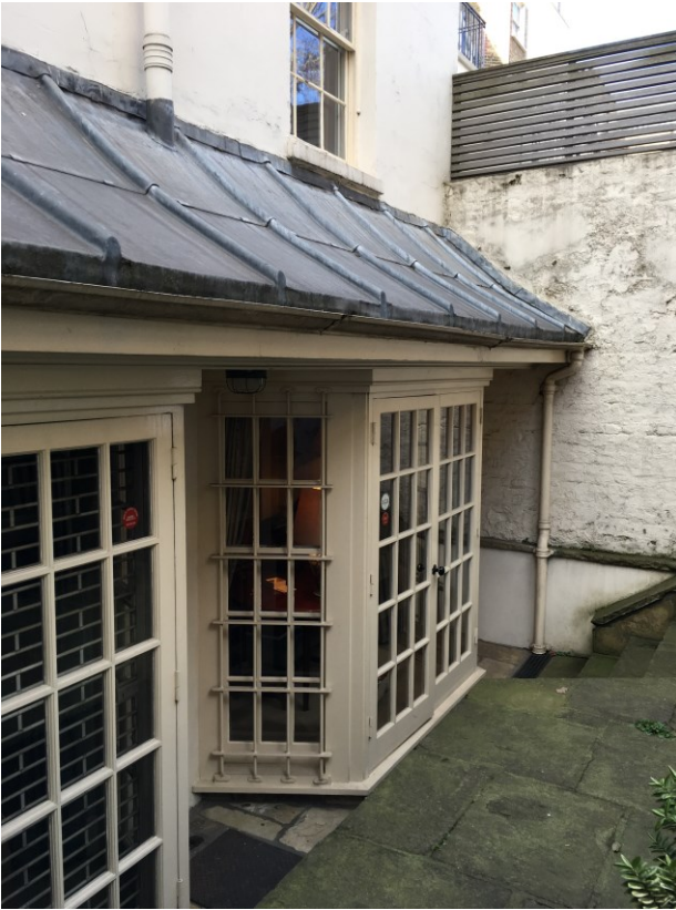
1 View of Courtyard to rear, showing modern bay windows and associated lead roof
