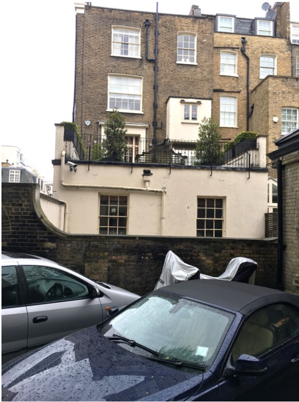
1 View of rear elevation from St. Peter's churchyard
