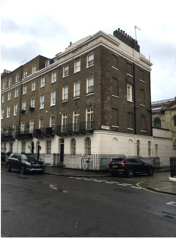
1 View of house from Wilton Street
