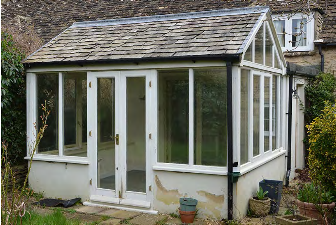
Plate 11 Boxwood Cottage rear extensions
