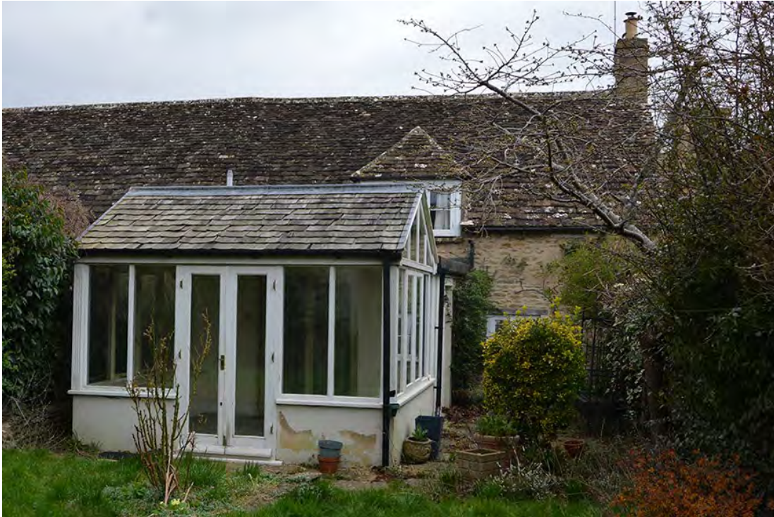
Plate 3 Boxwood Cottage rear elevation from the south east
