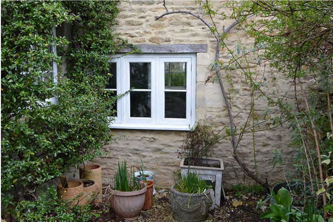
Plate 14 Boxwood Cottage rear elevation window proposed to be changed to doorway
