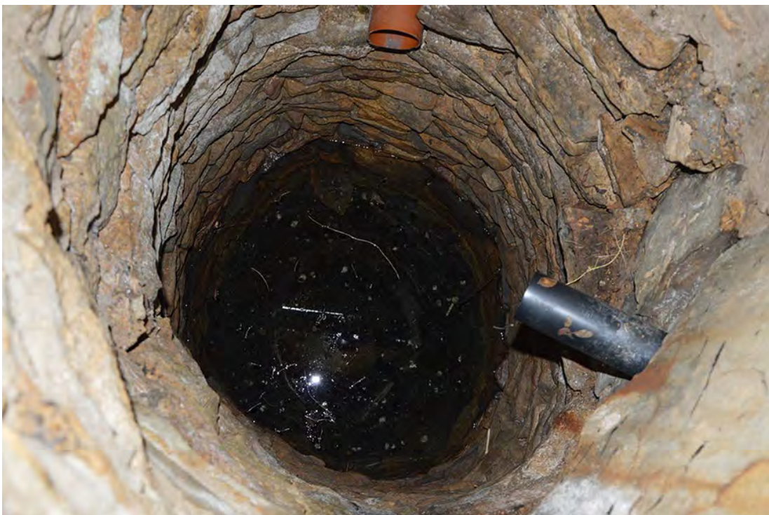
Plate 6 Boxwood Cottage well interior
