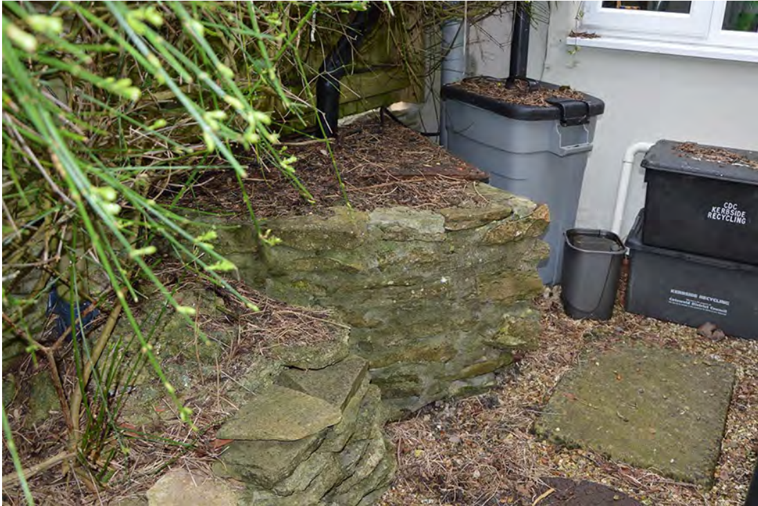
Plate 5 Boxwood Cottage well from the south east
