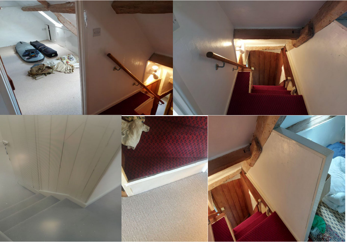
Existing first floor staircase including door opening and internal timber panelling.
