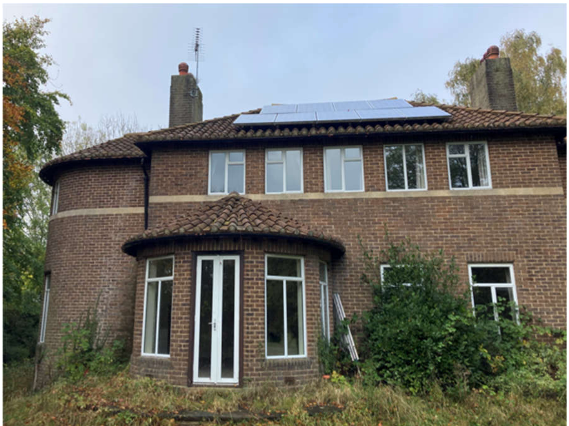
Figure 3: The vicarage southeast facing rear elevation
