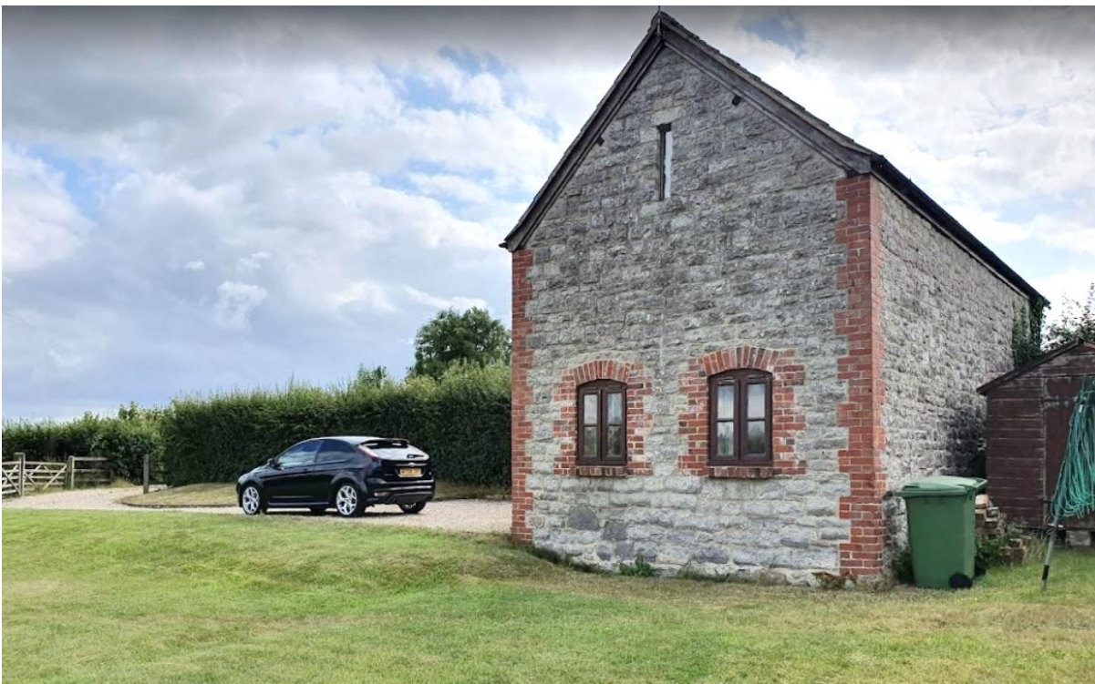
Top: Existing converted barn, parking area and lawns – south elevation Below: Converted barn and driveway– east elevation
