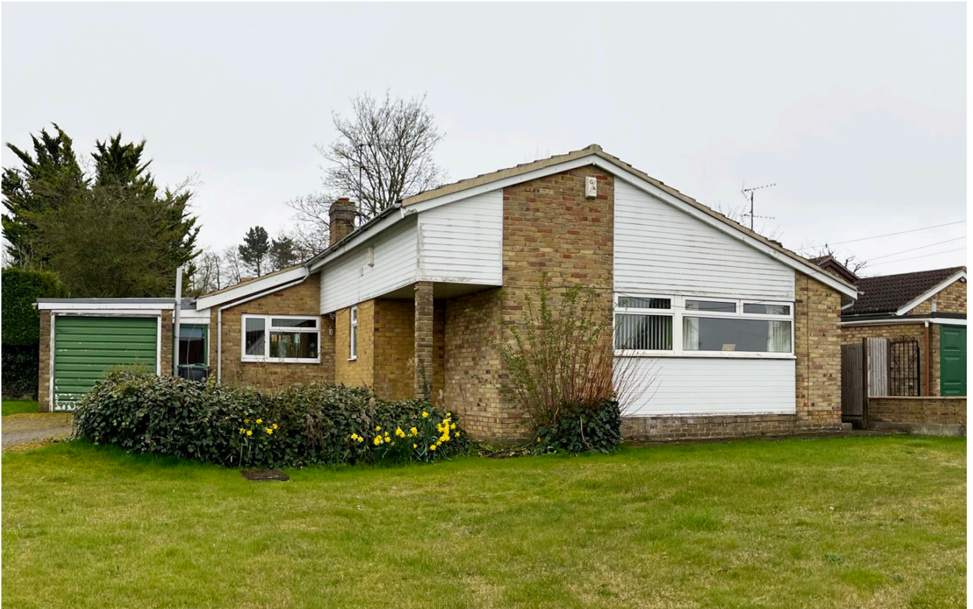
1. Existing front view
