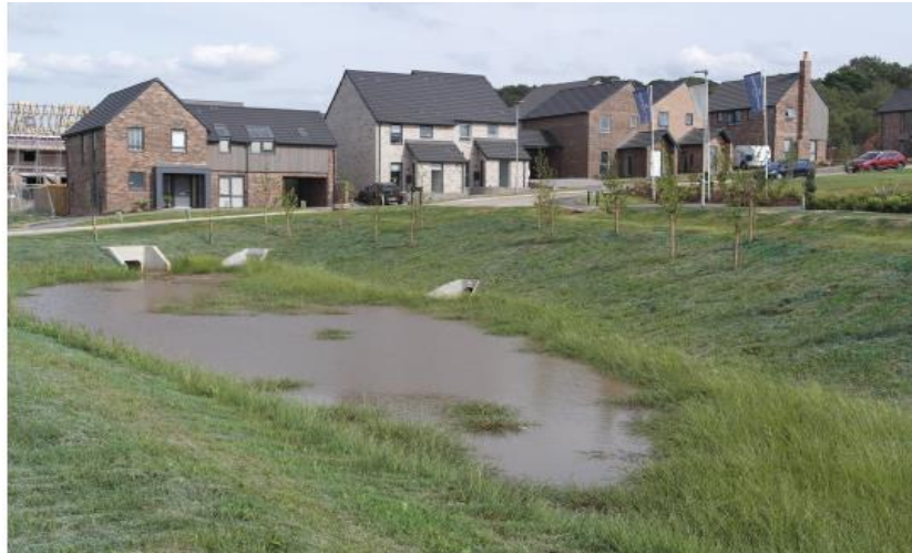
Figure 2-g: Example of a typical detention basin.
