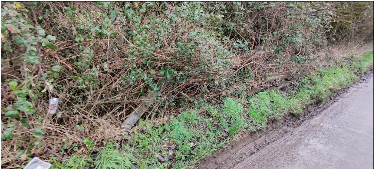
Figure 11 - Blocked Culvert at Vicarage 2
