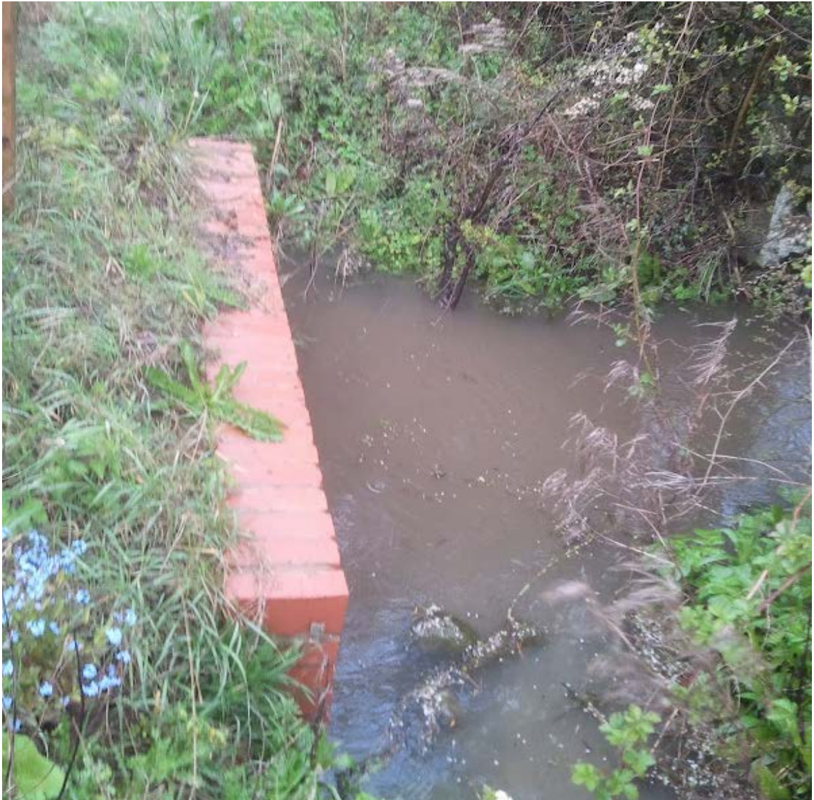
Figure 2.9 Parish Council Photo Carpenters Arms Culvert
