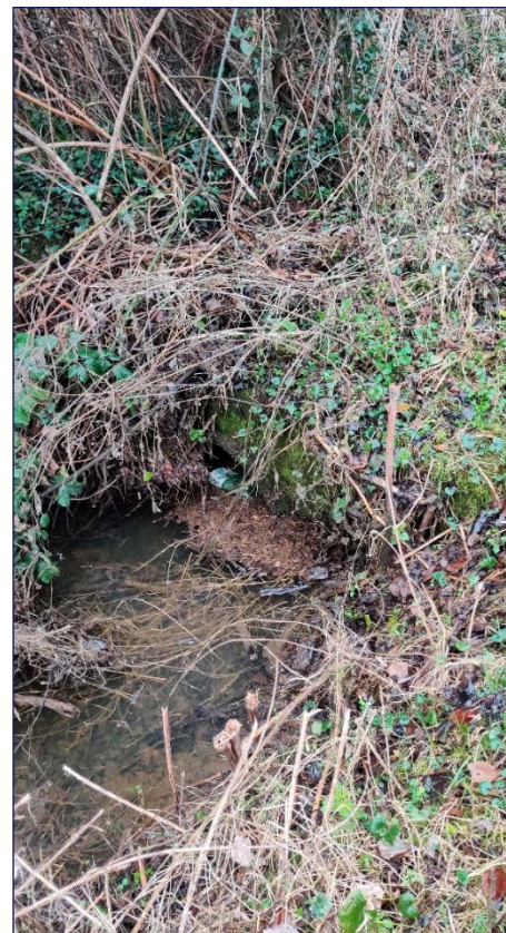
Figure 5 - Rowborough Culvert Outfall
