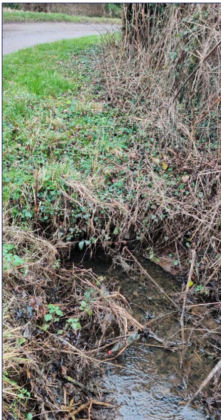
Figure 4 - Rowborough Culvert Inlet
