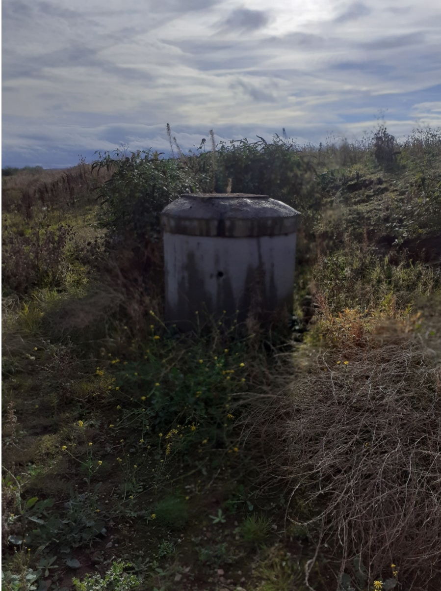
PLATE 5 – RASIED MANHOLE ALONG THE WESTERN BOUNDARY
