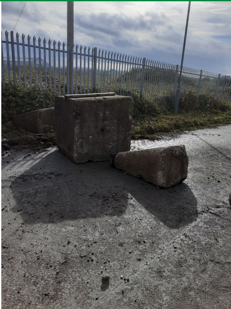
PLATE 1 – CONCRETE BLOCKS ACROSS ACCESS ROUTE
