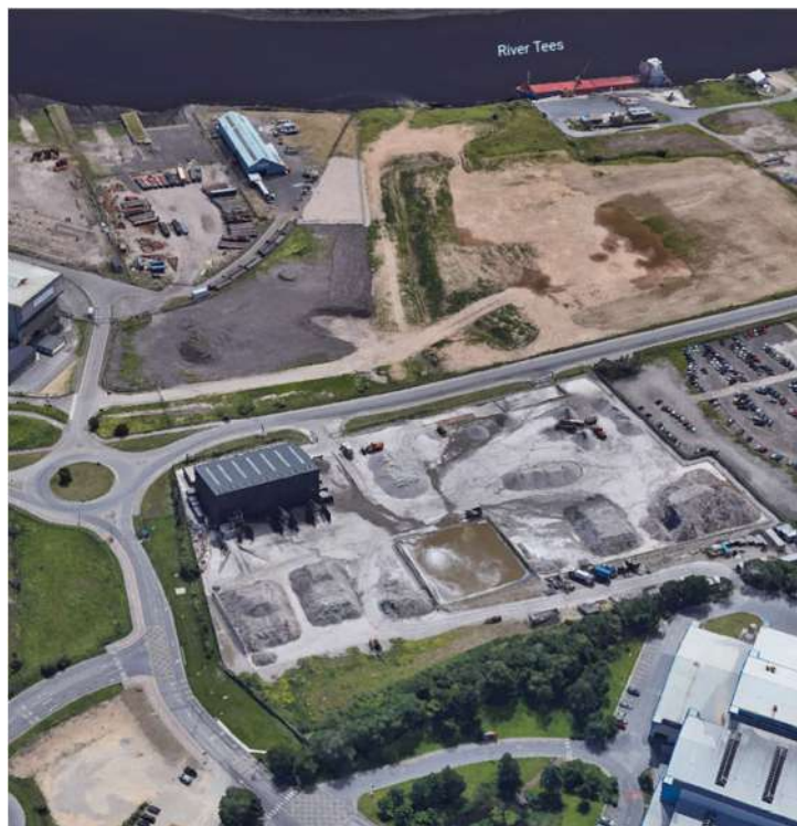
Aerial view of site from the north
