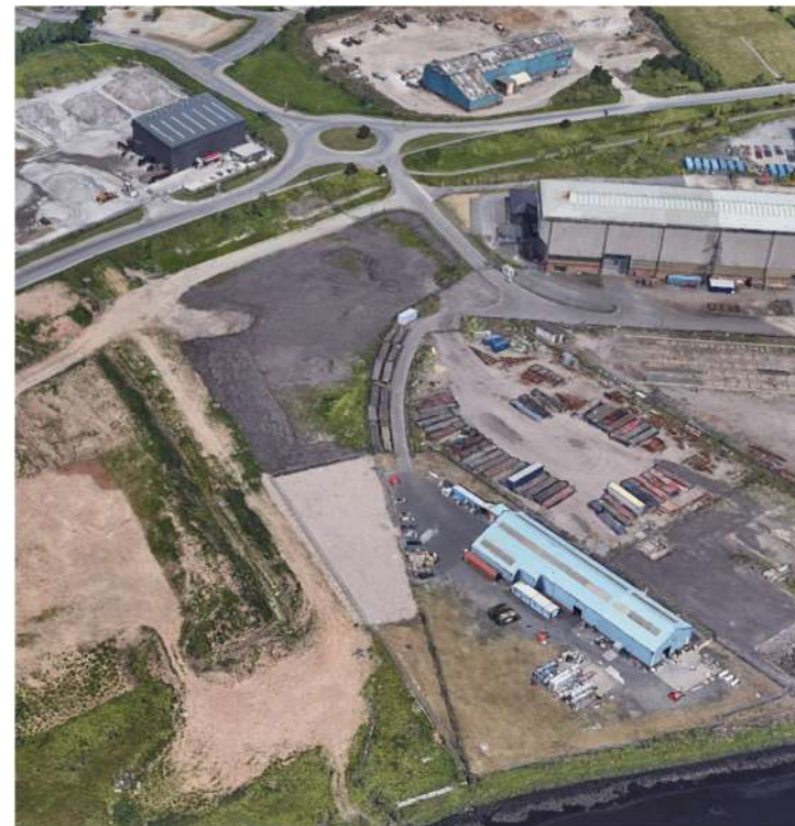
Aerial view of site from the south
