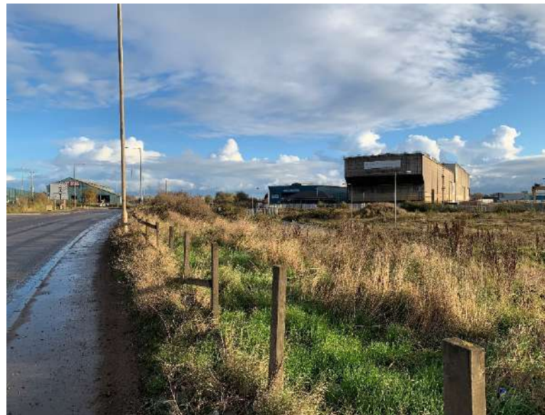
View East from A1046 Haverton Hill Road showing existing buildings on adjacent site
