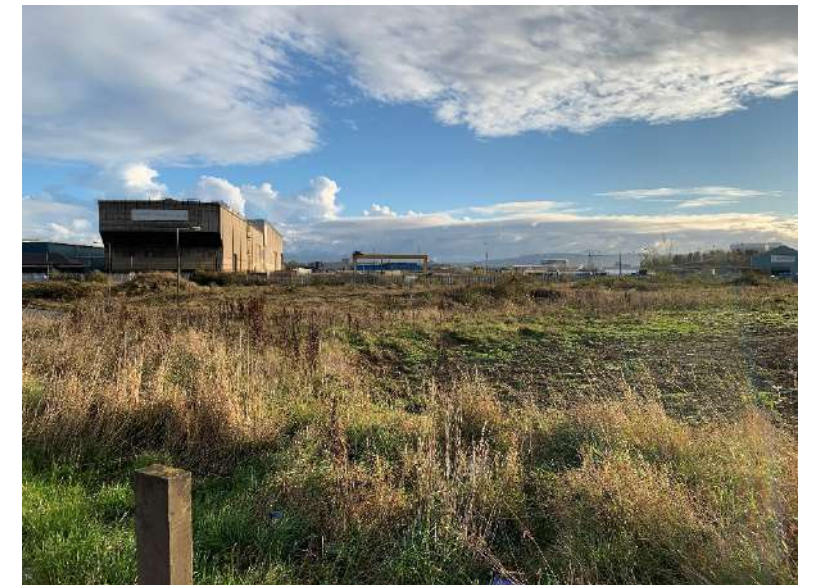
View South East from A1046 Haverton Hill Road showing existing buildings on adjacent site
