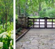
New entrance gates and posts. Slightly widened to 3.6m and set back. - Whin edging setts taken up and reused to line the entrance gate strip. - Purple beech outside of gates along
