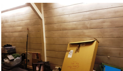
View of interior of office timber frame.
