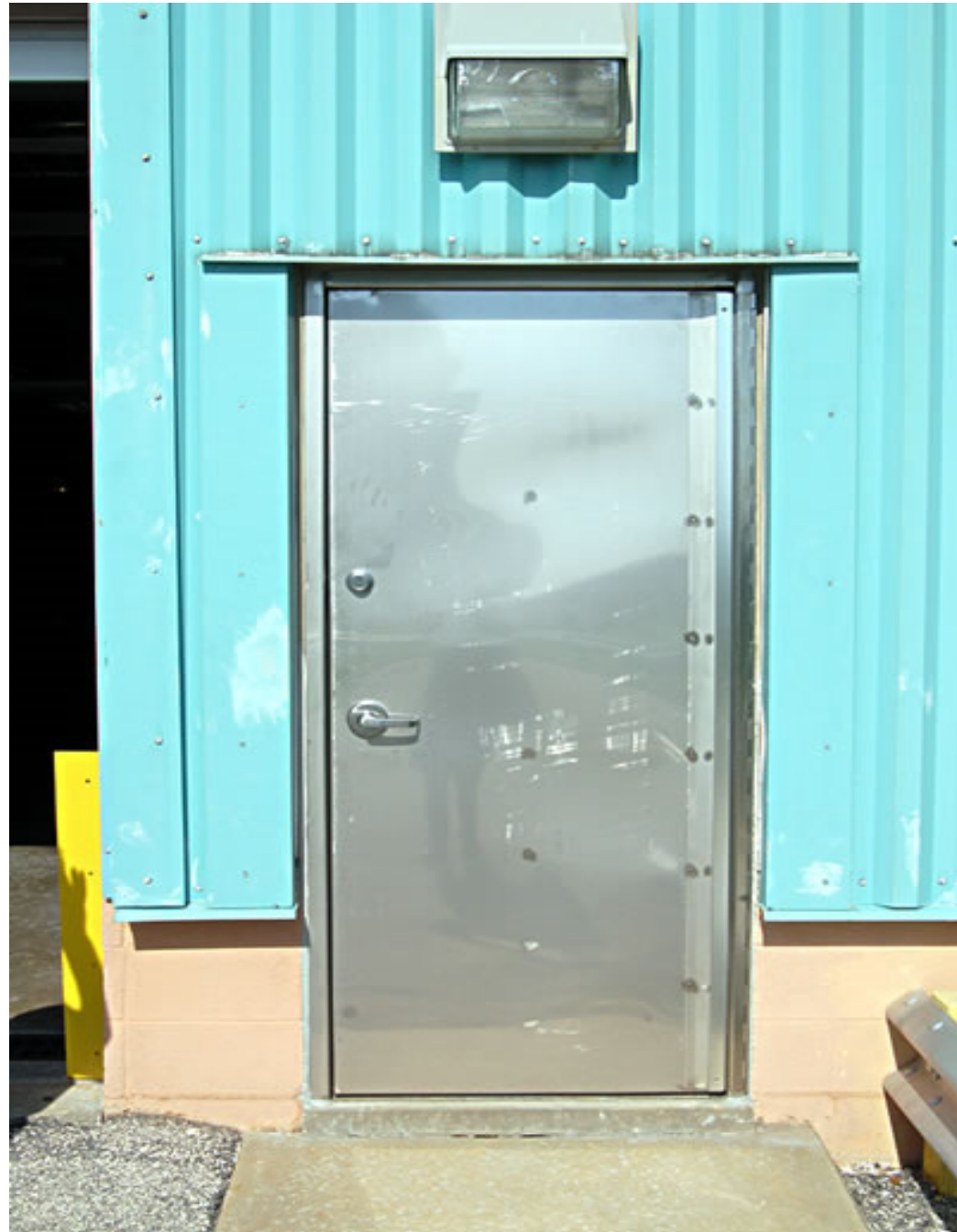
FIGURE 24 –PEDESTRIAN FLOOD DOORS
