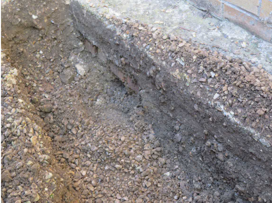
PHOTO No. 10 – TRIAL HOLE EXPOSING CONCRETE RAFT SLAB AND SUB-BASE
