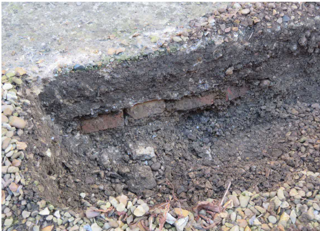
PHOTO No. 11 – TRIAL HOLE EXPOSING CONCRETE RAFT SLAB AND SUB-BASE
