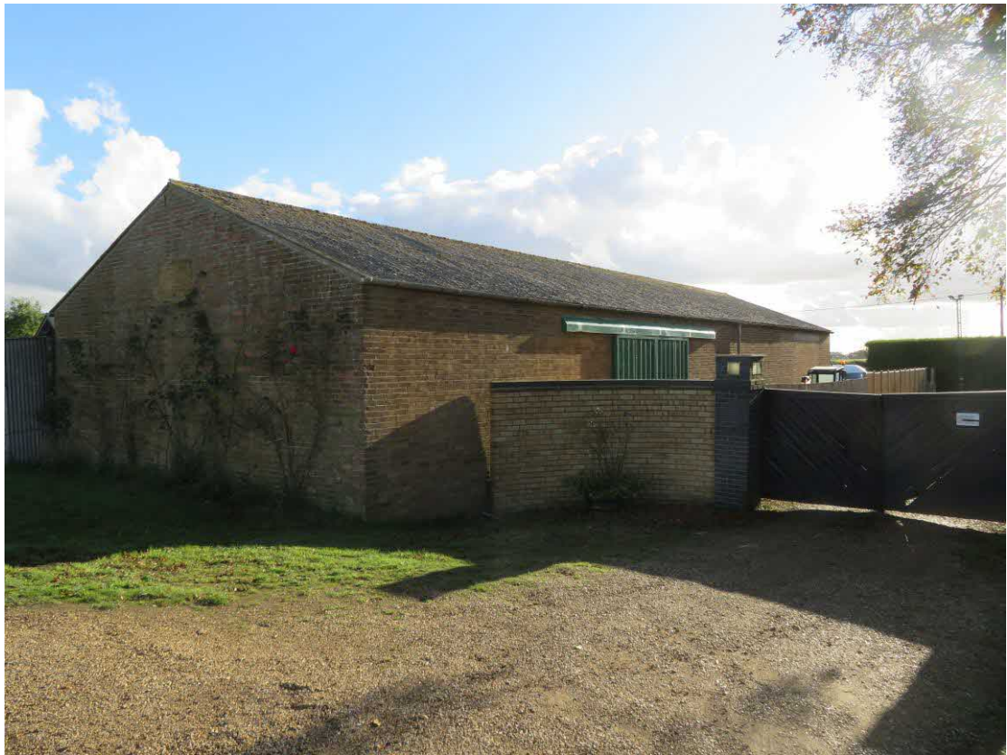
PHOTO No. 2 – NORTH WEST ELEVATION
