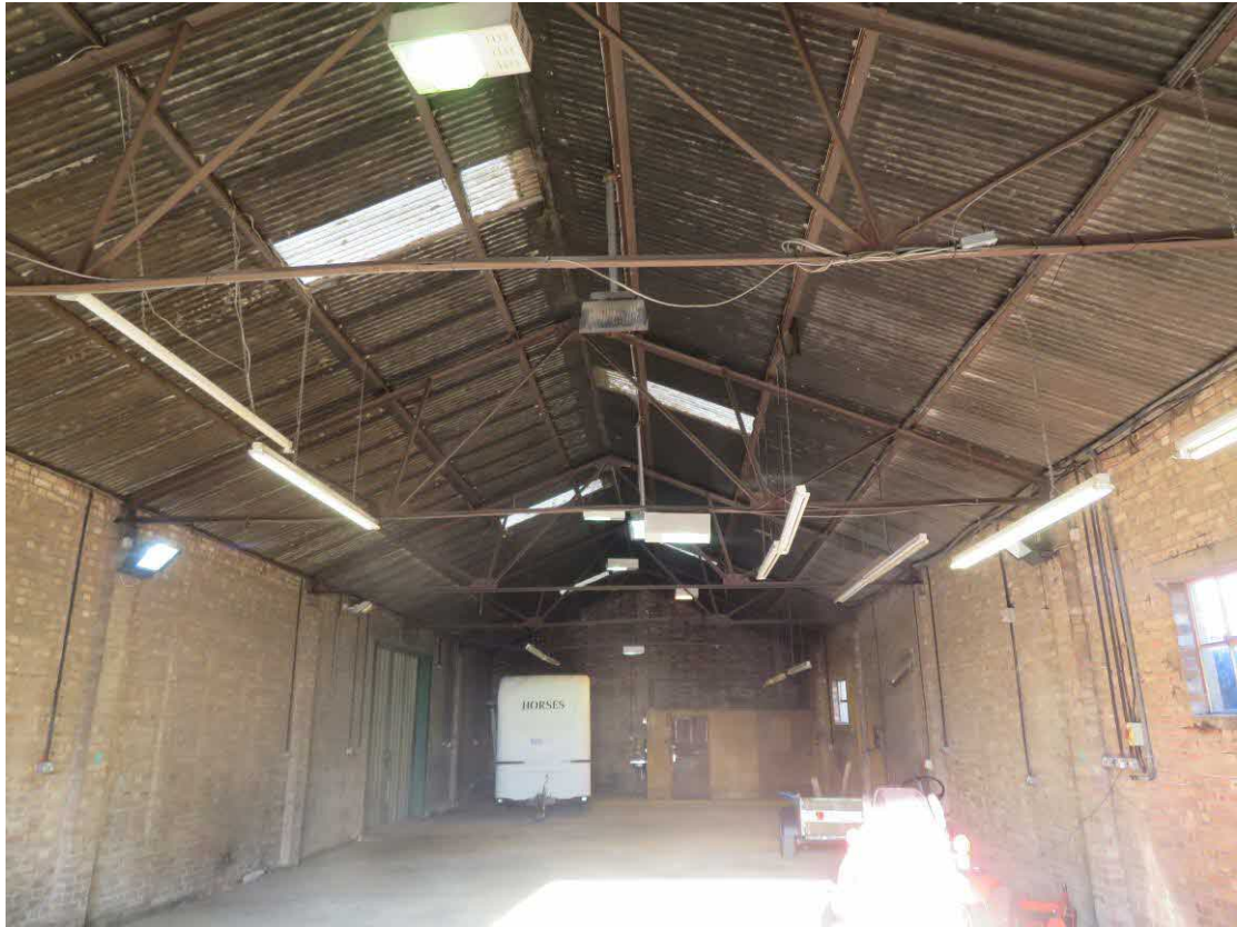
PHOTO No. 5 – INTERNAL ROOF TRUSS ARRANGEMENT WITH SUPPORTING PIERS
