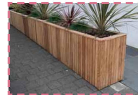
Removable planters defining edge of terrace. Height to match mews house planter heights and finish stained to match timber panels on facade.
