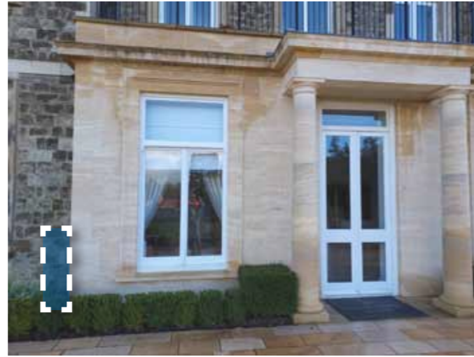
Apartment 13 - External socket & switch location on facade
