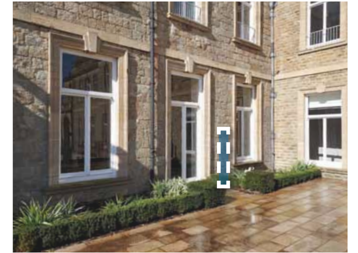
Apartment 15 - External socket & switch location on facade
