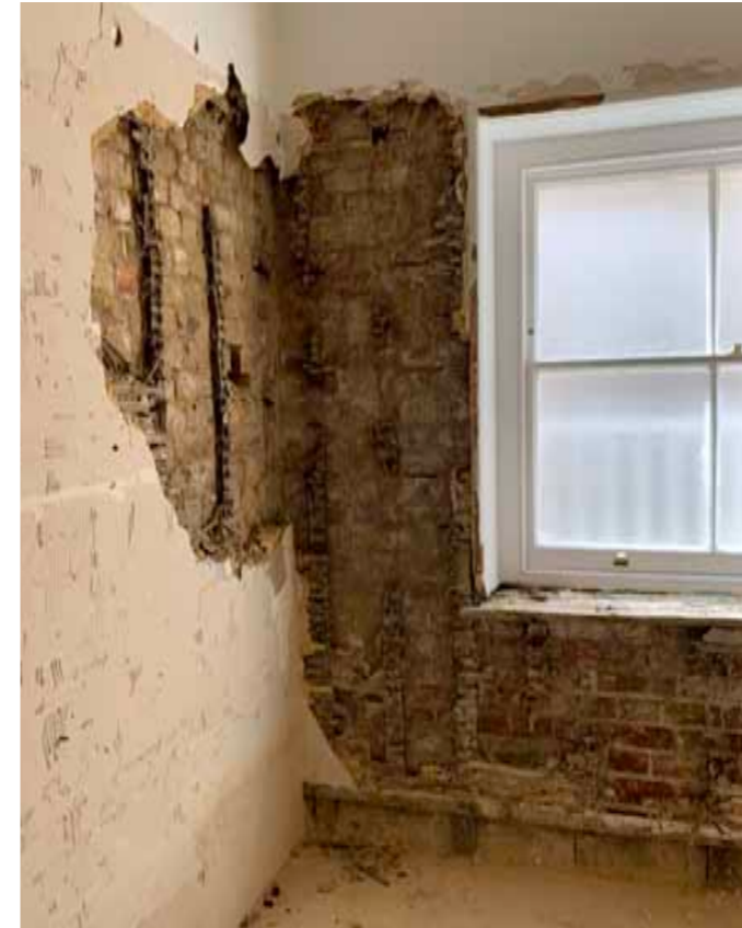
Apartment 19 bathroom after removal of wall tiles
