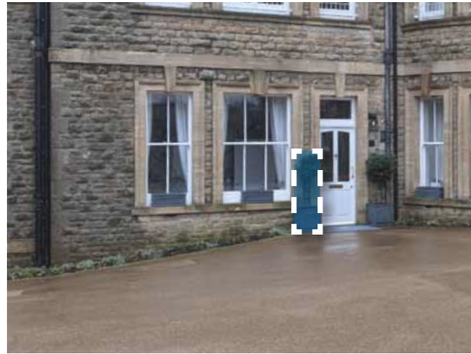
Apartment 12 - External socket & switch location on facade
