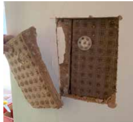
Plaster directly onto the solid wall with no insulation
