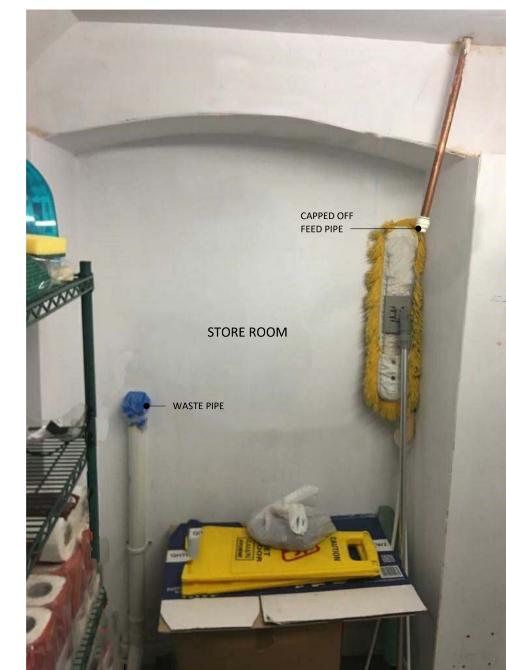
6 Store Room Photo 1 : 20
