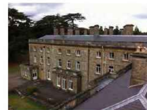
East elevation of the 18th century building from the roof of the late 19th century extension
