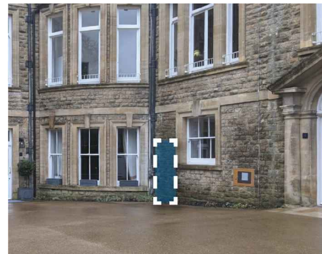
Apartment 11 - External socket & switch location on facade
