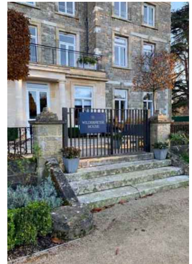
V1. Existing apartment 13 access
