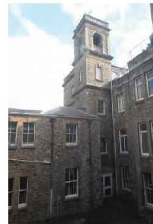
Internal courtyard, late 19th century and extension, looking south-east
