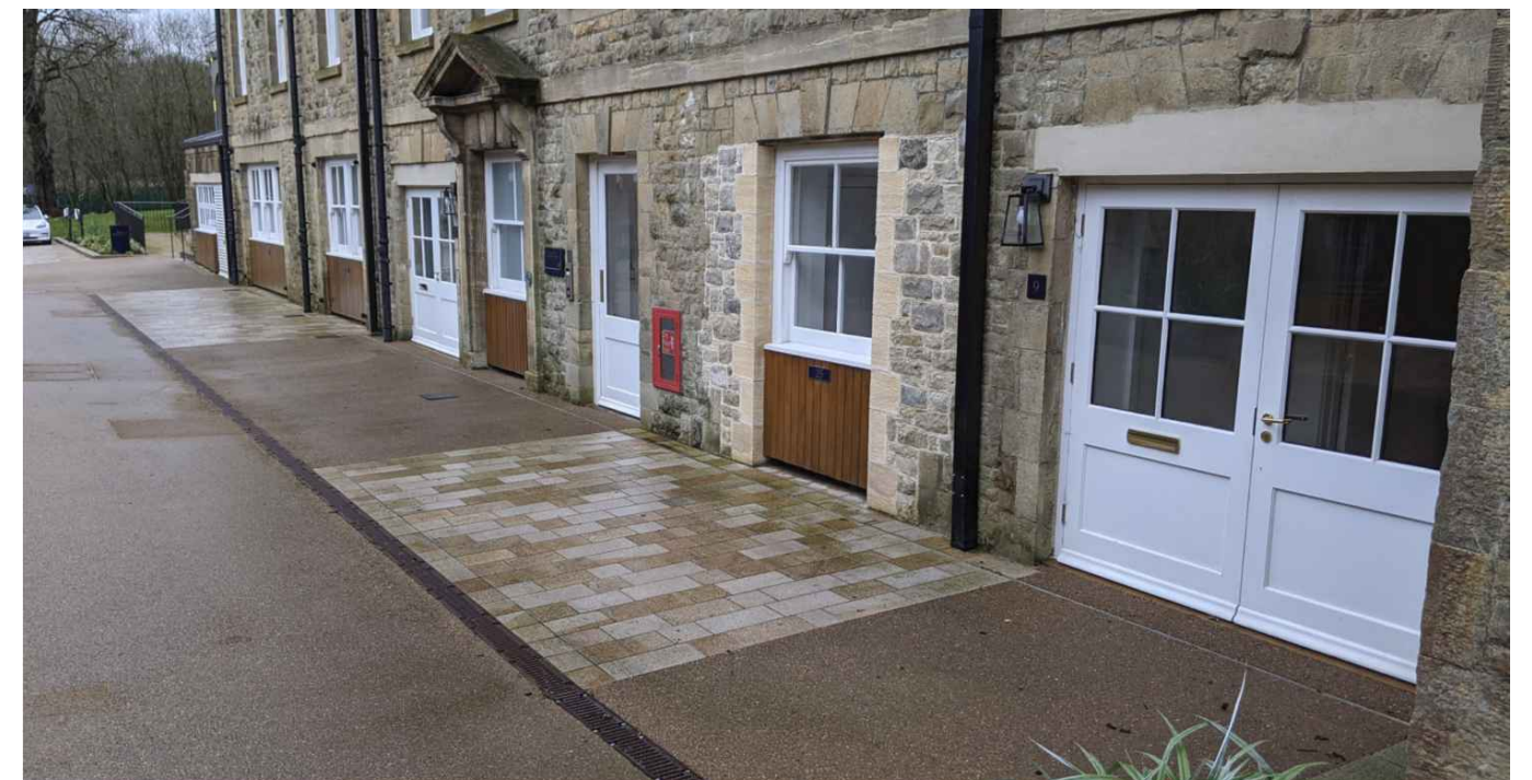
Apartments 9 and 10 entrances with parking against facade and no buffer entrance zone.
