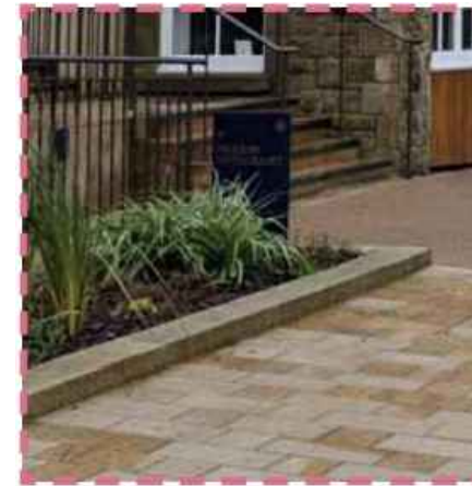
Removable planters defining edge of terrace. Height to match mews house planter heights and finish stained to match timber panels on facade
