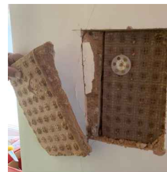
Plaster directly onto the solid wall with no insulation
