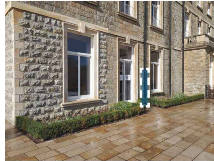
Apartment 14 - External socket & switch location on facade
