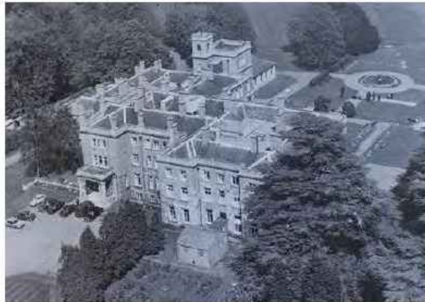
Aerial photograph showing the west elevation in 1960 showing extension against 18th century main entrance. This extension was replaced with another extension during the late 20th century (still extant)
