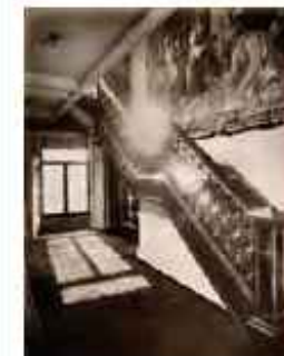
Interior view showing the ebony staircase at The Wildernesse, 10th July 1889
