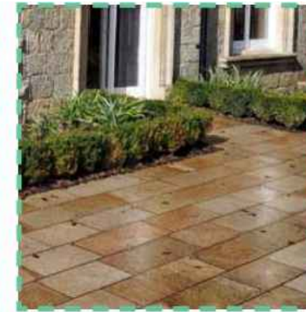
Terracing to apartment 13, 14, and 15 use rectangular pavers to define terrace areas. These will be used in a similar fashion to apartments 9 & 10.
