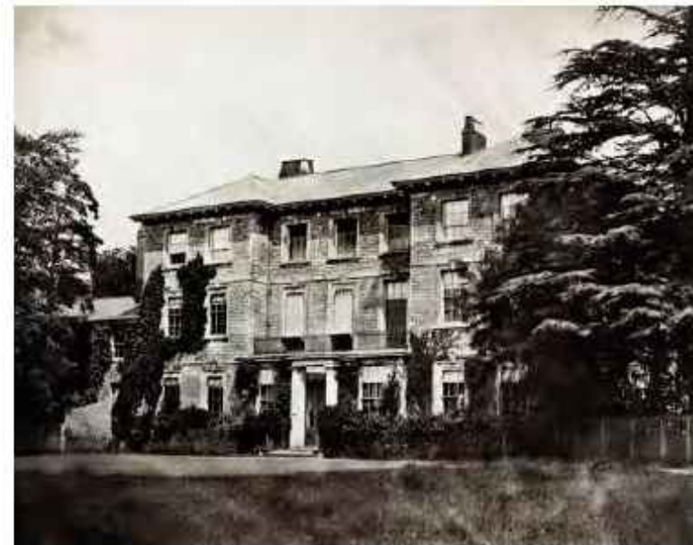
Exterior view of entrance (west) front, 1860-69
