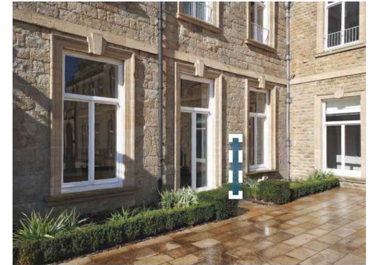
Apartment 15 - External socket & switch location on facade
