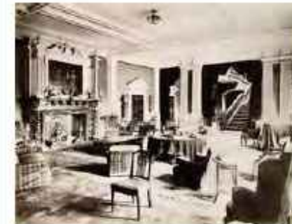
Interior view of the hall at The Wildernesse, 10th July 1889
