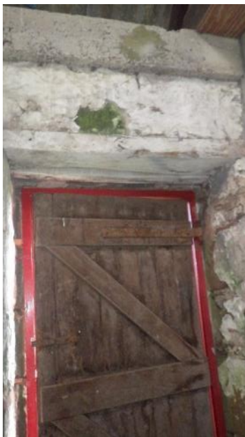
Photo 15: Doorway with lintel providing roosting potential
