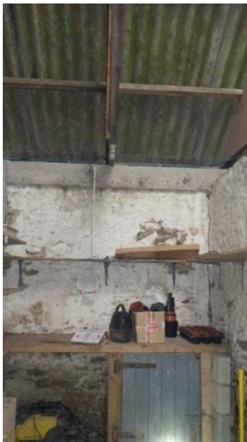
Photo 9: East view of room 1
