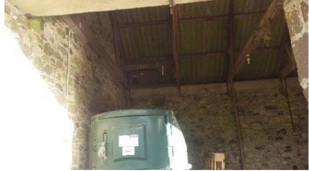
Photo 18: Internal view of woodstore
