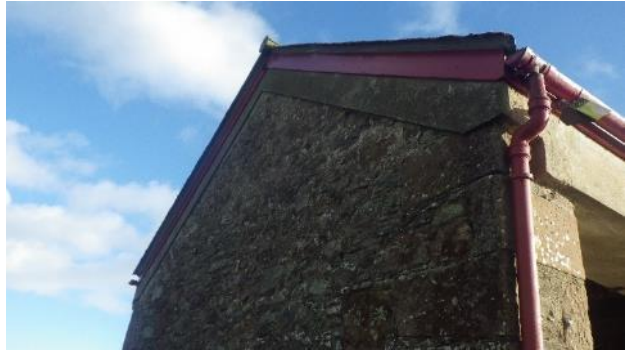
Photo 2: Southern gable end tightly sealed at wall head
