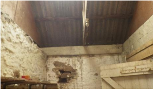
Photo 7: West view of room 1
