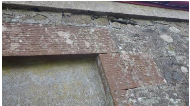
Photo 6: Crevices along eastern aspect
