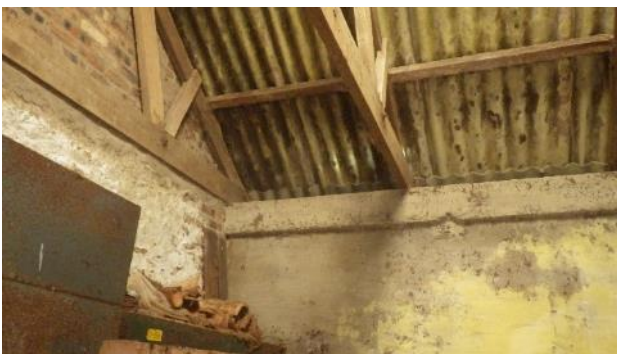
Photo 13: Eastern wall of room 2 (oil tank visible)
