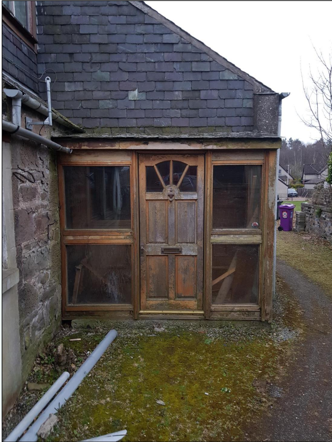
Figure 5. Vertical slates with no bat roost potential
