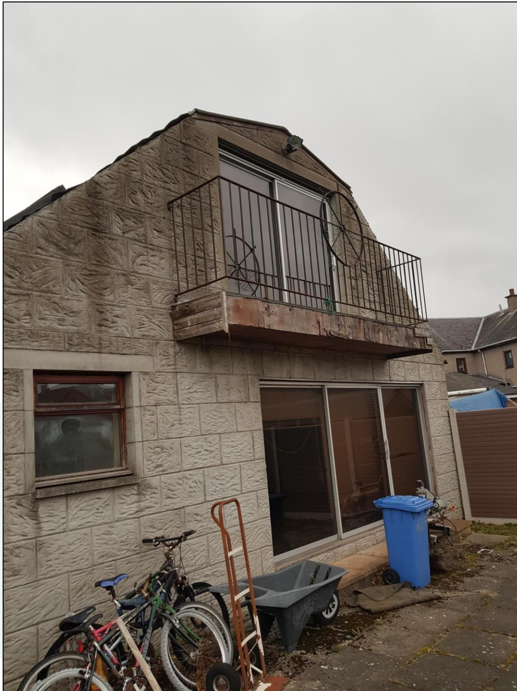
Figure 6. Stonework with no wall cavities present and no bat roost potential
