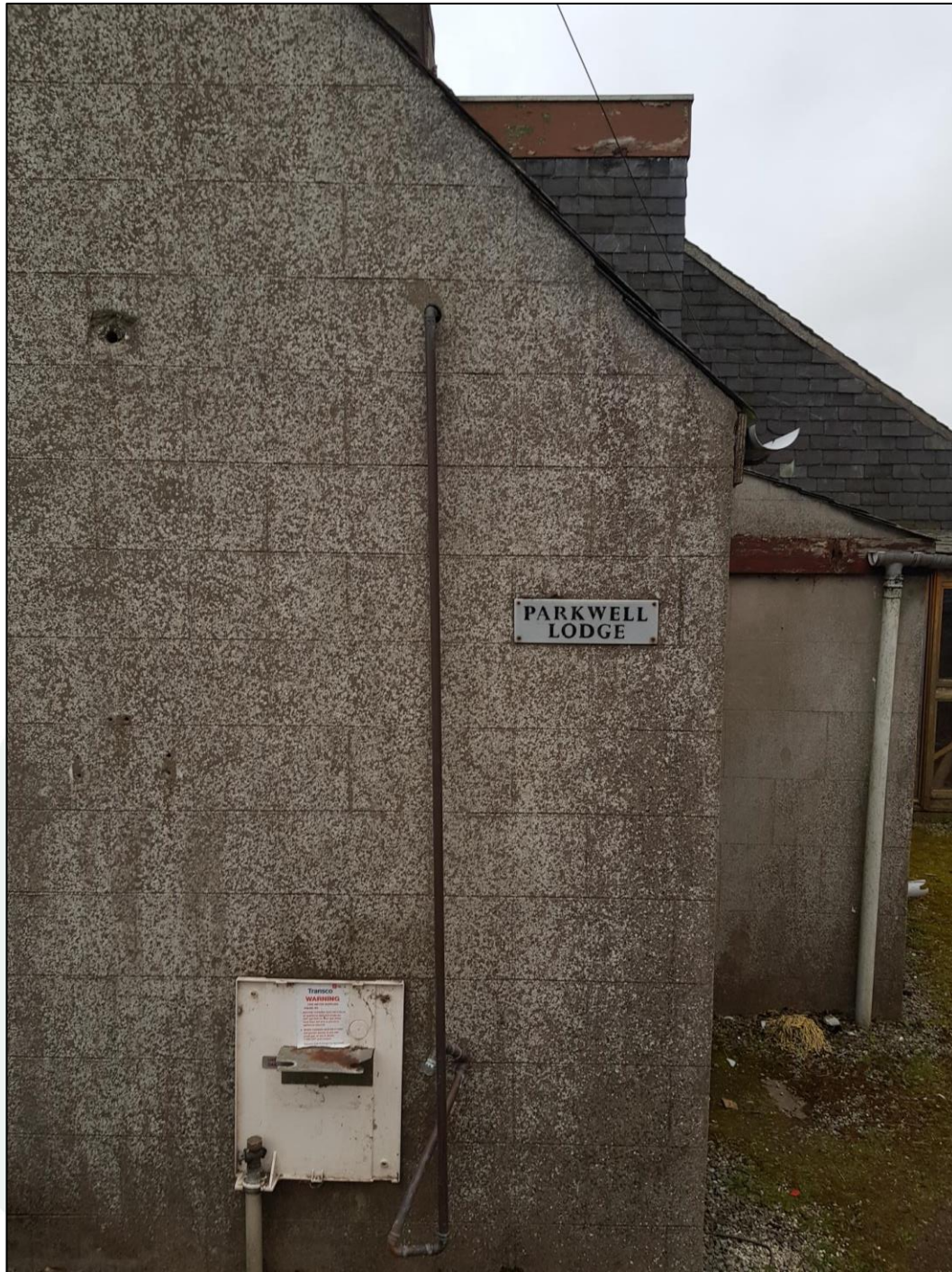
Figure 4. Stone gable ends with no bat roost potential.
