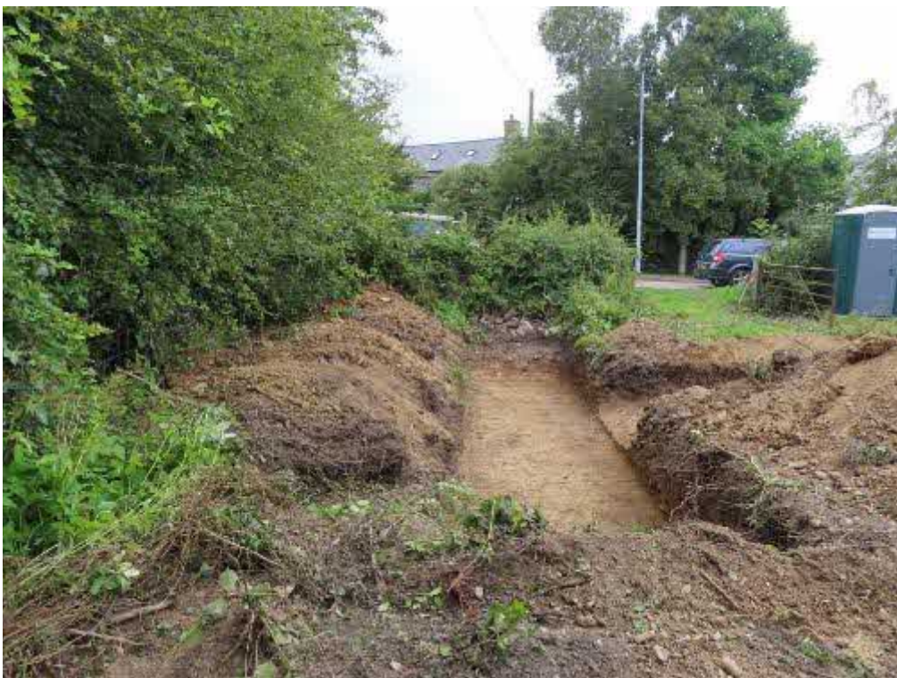
Photograph 4. View within the southwest boundary (left). Looking northwest from southeast.
