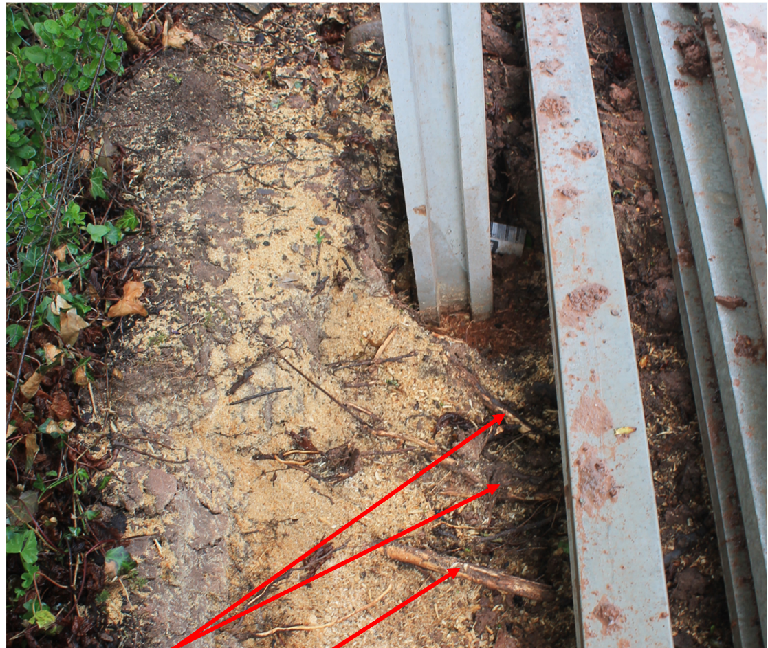
Trim back severed roots and retain large root (40mm diameter) intact, back fill with topsoil
