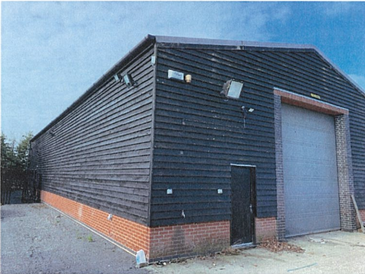
North East corner of the barn
