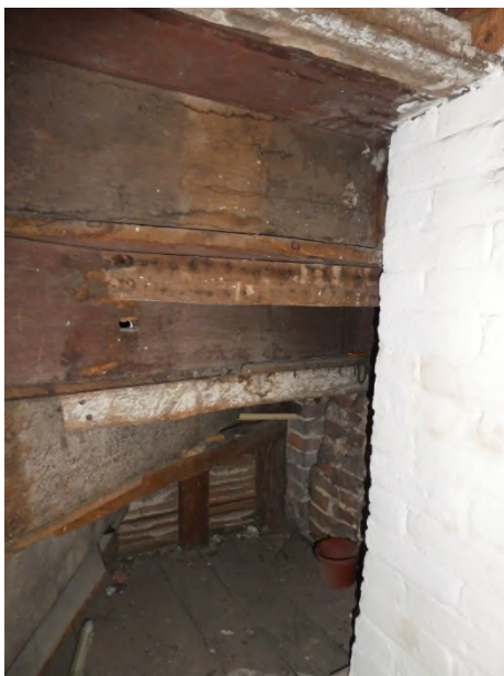
Figure 34: Staircase structure to the rear of F8
