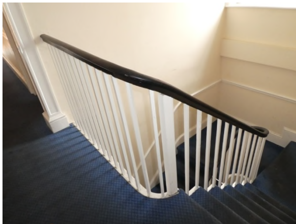
Figure 32: Early 19 th century staircase
