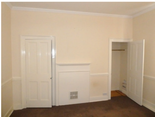
Figure 29: Blocked fireplace and cupboards in F5
