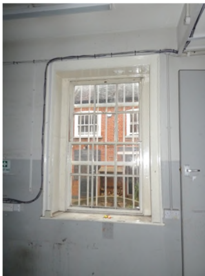
Figure 16: Sash window on the eastern side of G4
