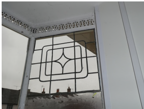
Figure 7: 20 th century glazing and 19 th century detailing
