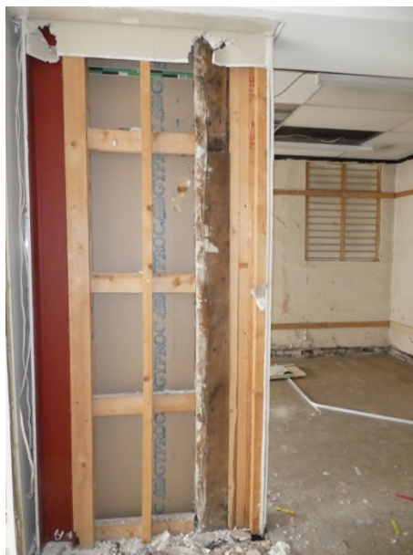
Figure 8: Timber post concealed behind a modern plasterboard finish
