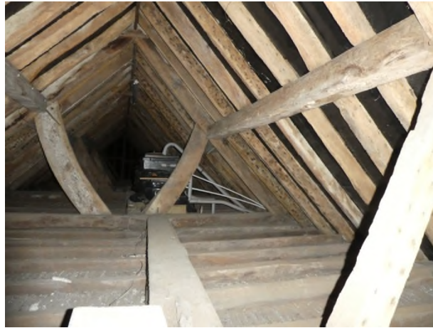
Figure 38: Roof structure over the western side of the rear wing
