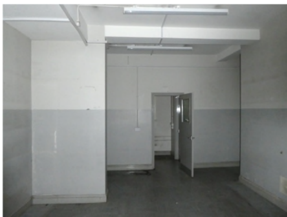
Figure 17: Short section of masonry wall (left) in G4
