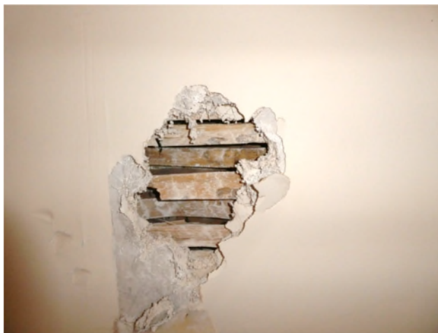
Figure 27: Riven lath and plaster finish associated with the cupboard on the north side of F3
