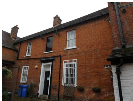
Figure 5: East elevation of 108 High Street
