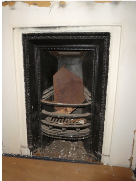
Figure 36: 19 th century register grate in F9
