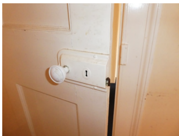
Figure 31: Metal rim lock with Bakelite door knob to F6
