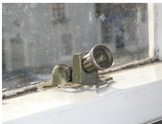
Figure 21: Detail of a Brighton pattern sash fastener
