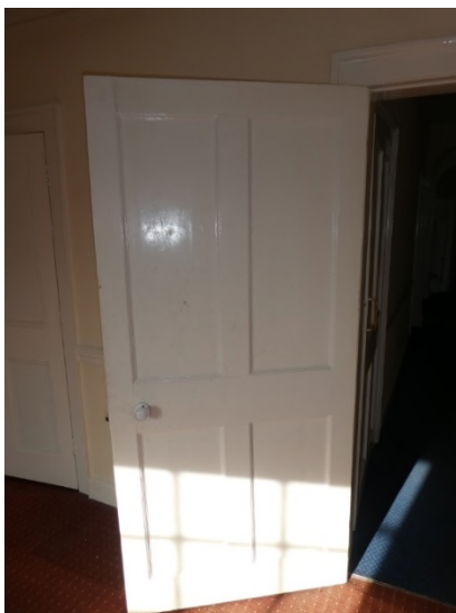
Figure 20: 4-panelled door to F1
