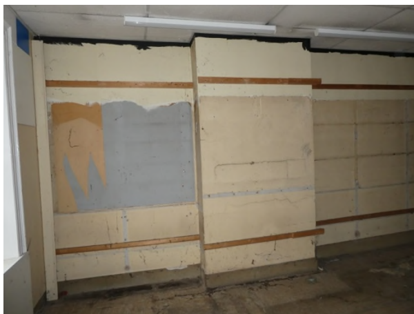
Figure 12: Chimney breast on the western side of G1
