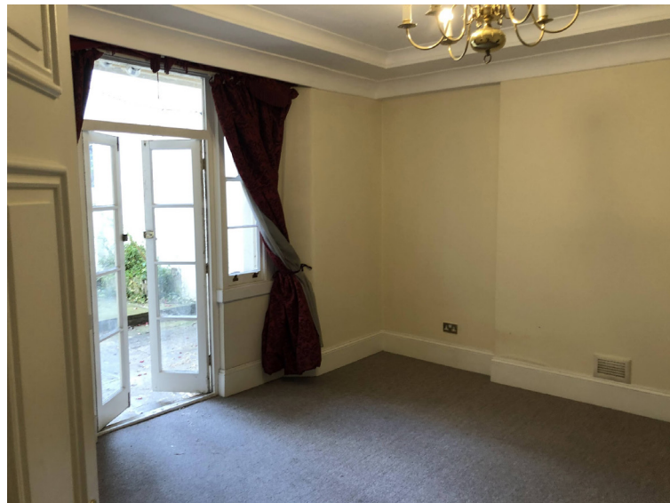
Plate 7 Showing ground floor room and patio doors to be removed for the extension. Note these doors are later additions.
