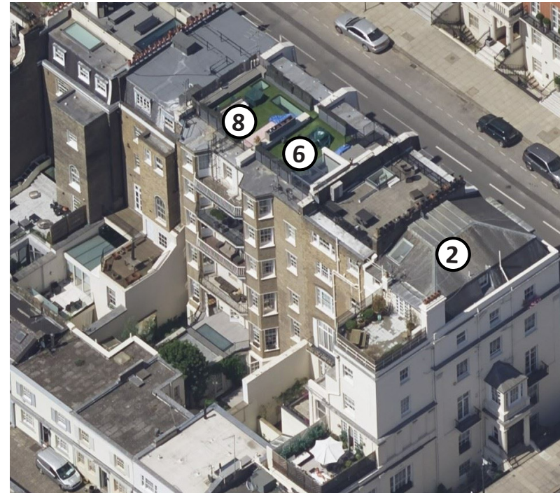
Figure 9 Oblique aerial view of the listed terrace showing properties with side extensions to the rear.
