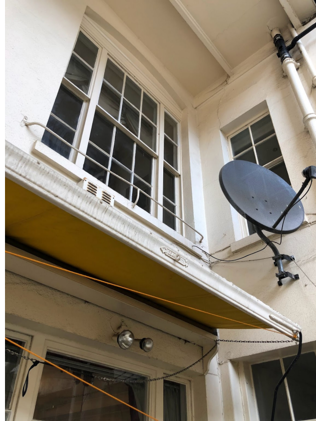
Plate 4 Showing disjointed appearance of the rear and unsympathetic awning above lower ground floor.
