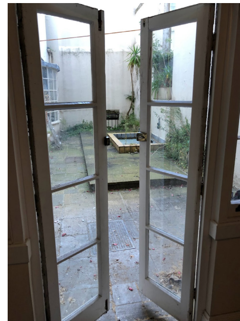
Plate 8 Detail of modern patio doors to be removed
