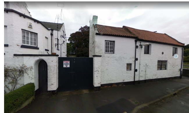
The black gate forms the secluded access to car charger
