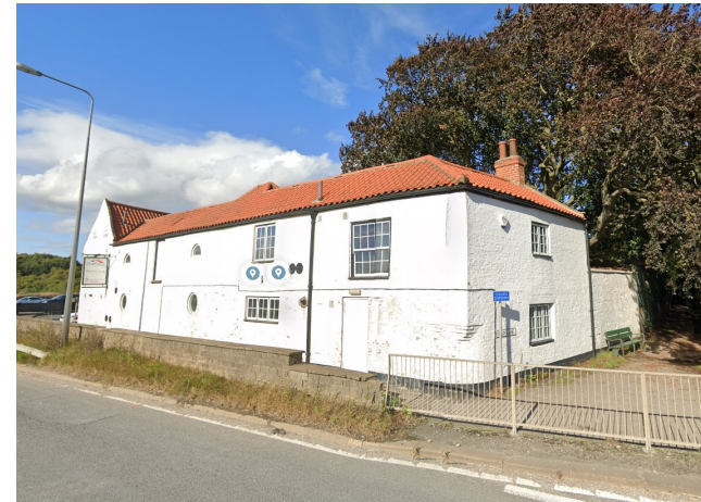
A view of the Old Foundry from the A63 Highway
