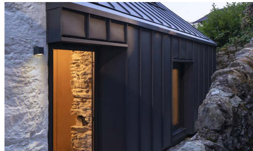
Standing seam coated steel cladding - proposed colour Anthracite RAL 7016
