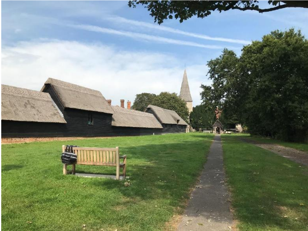
Figure 21: Church of St John viewed from The Street to the south
