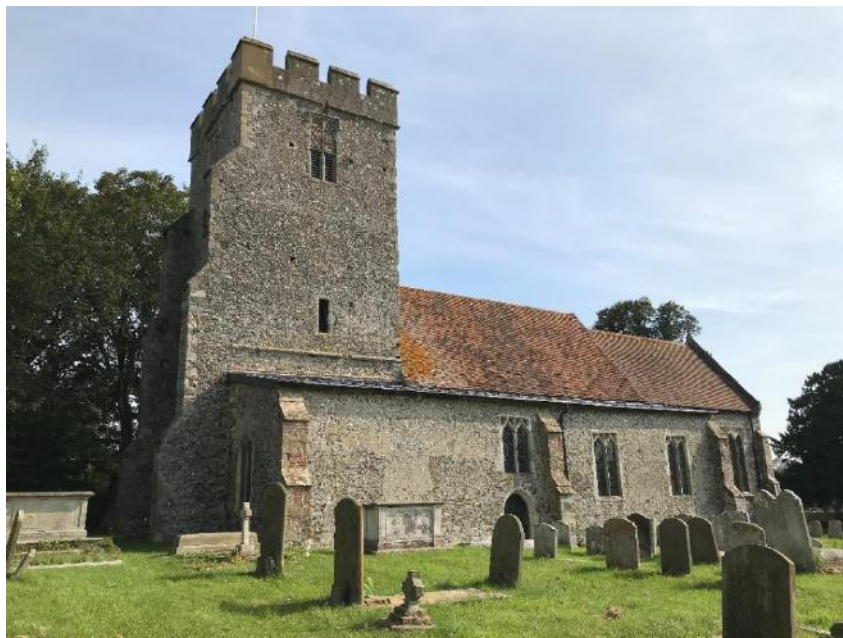
Figure 27: Church of St Andrew, Wickhambreaux, viewed from the south
