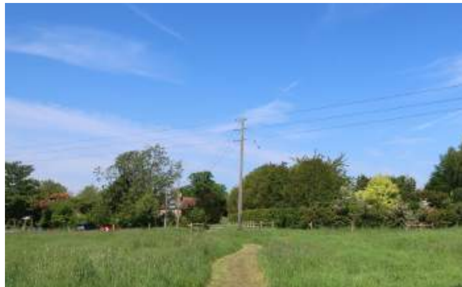
Orchard with electrical infrastructure overhead
