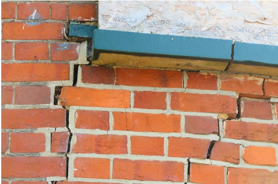
Photo 8 , cavities within brickwork provide roosting features and access points for bats.
