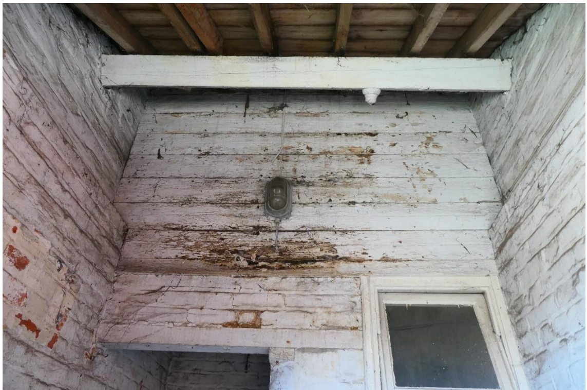
Photo 5 , internal view of section C, looking east.
