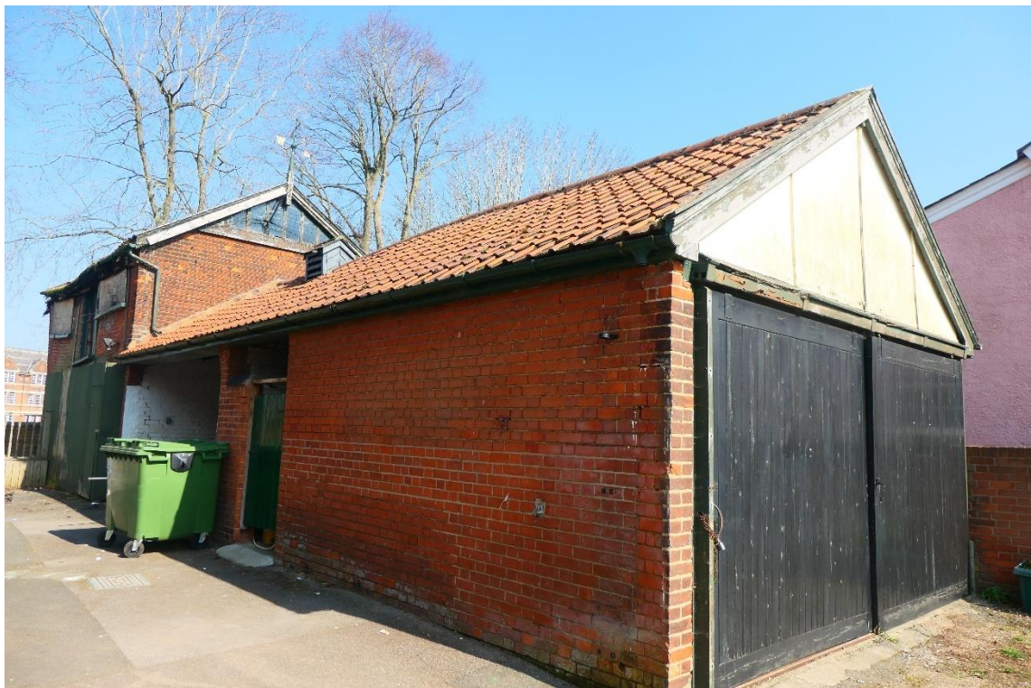
Photo 1 , south and west aspects of building one, looking northeast.
