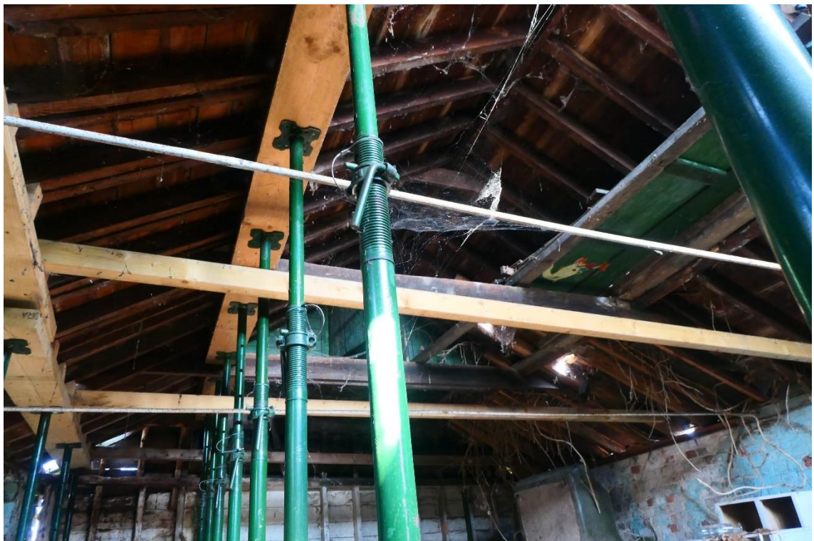
Photo 3 , internal view of Section A, looking north.
