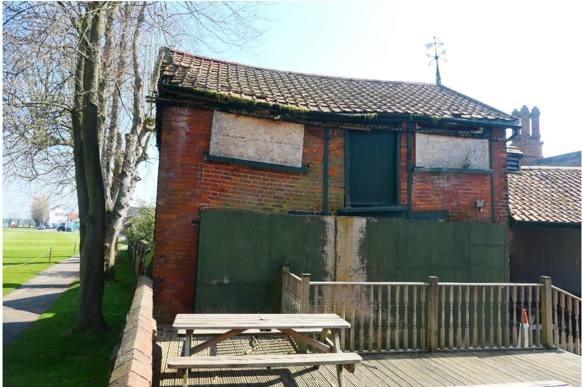
Photo 2 , north and west aspects of Section A, looking east.
