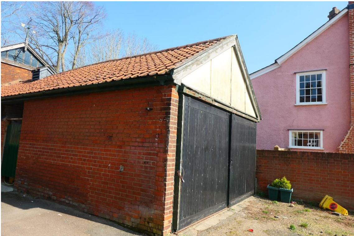
Photo 7 , south and west aspects of Section E, with internal access unavailable.
