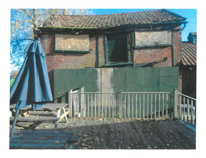
In order to make the building safe the roof of the building is back propped down on to the first floor, and the first floor then propped down to ground level. The decayed beam across the front opening has also been propped.
