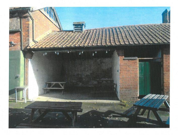
The roof pitches of the cart lodge have deflected as has the front beam over the opening. A study of the roof structure reveals that the original roof to consist of common rafters, purlins and collars. The purlins have deflected significantly
