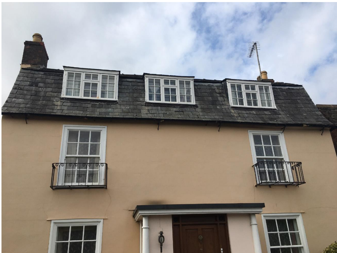
The first floor sash windows from The Burgage
