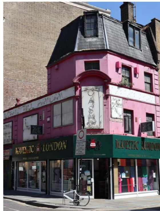
05 Photograph of Existing Facade Scale: nts
