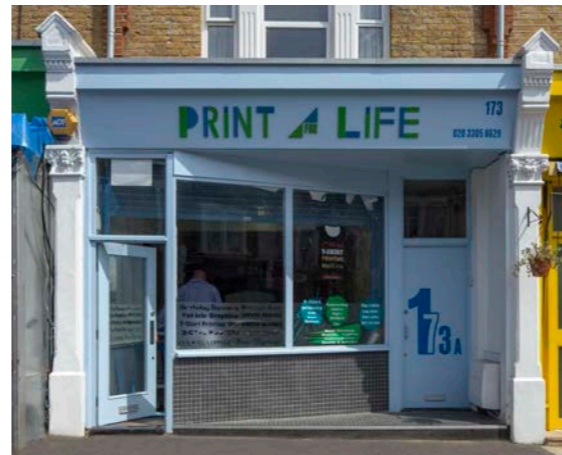
Console brackets and pilasters repaired and painted
