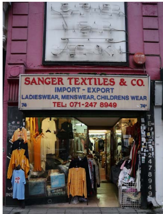
04 Photograph of Existing Facade Scale: nts
