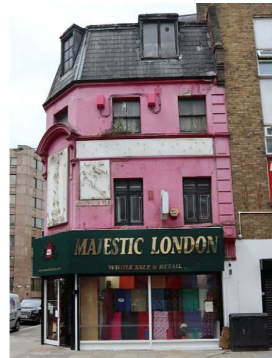
06 Photograph of Existing Facade Scale: nts
