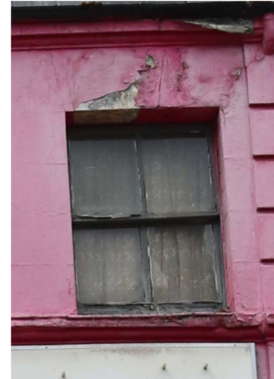
03 PHOTOGRAPH - Existing Dormer Window 1 Scale: Not to scale
