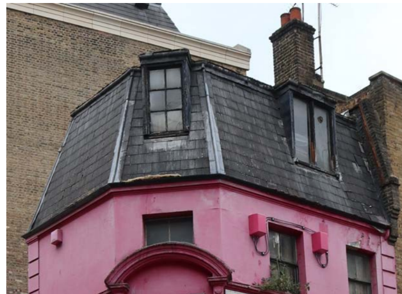
02 PHOTOGRAPH - Existing Roof Condition Scale: Not to scale
