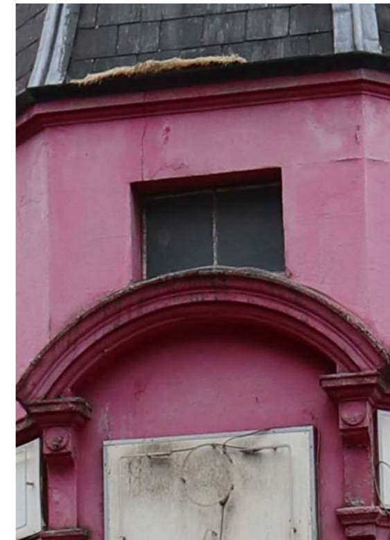
06 PHOTOGRAPH - Existing Dormer Window 2 Scale: Not to scale
