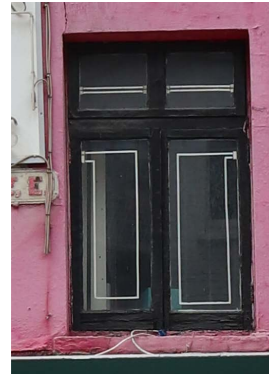
03 PHOTOGRAPH - Existing 1st Floor Casement Window Scale: Not to scale
