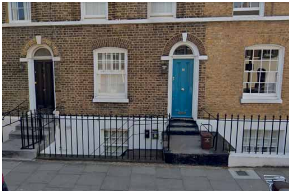
Railings and staircase to lower ground of No10 Aberavon Road
