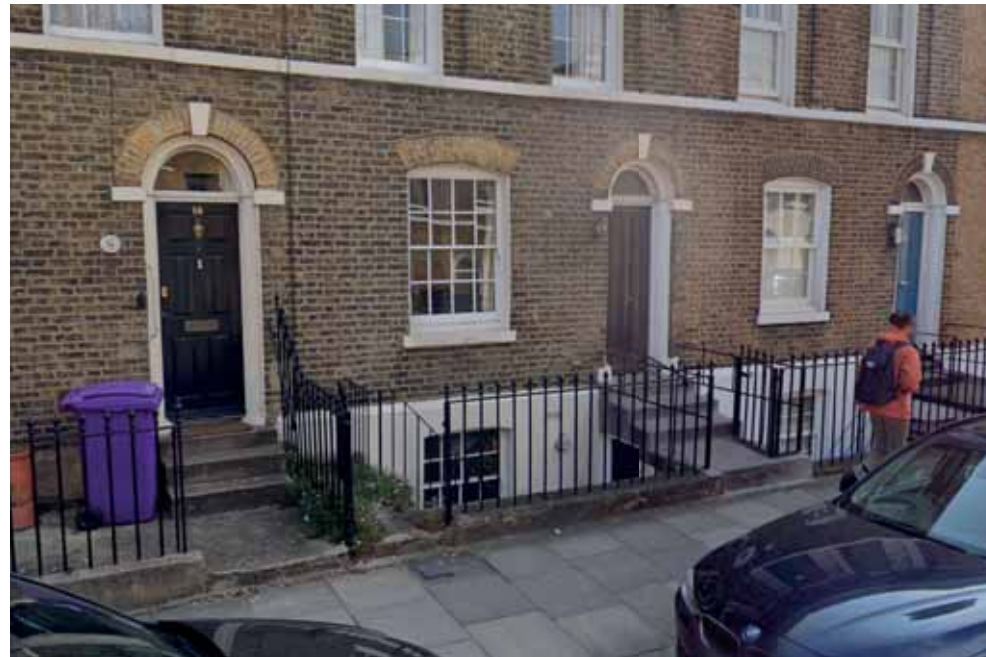
Railings and staircase to lower ground of No12 Aberavon Road
