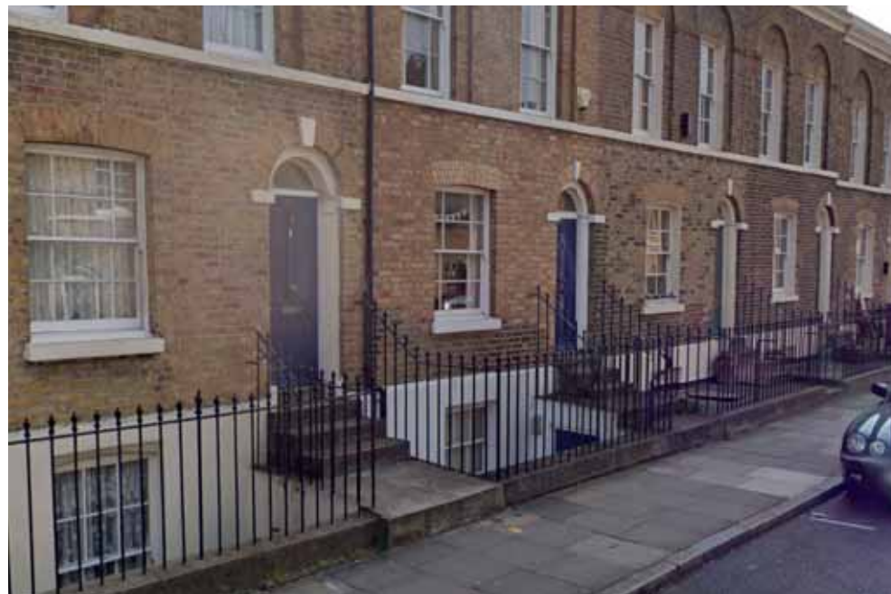
Railings to No26 and 28 Aberavon Road, with access to courtyard at lower ground level
