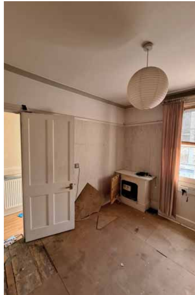
Existing Living Room (Upper ground floor)
