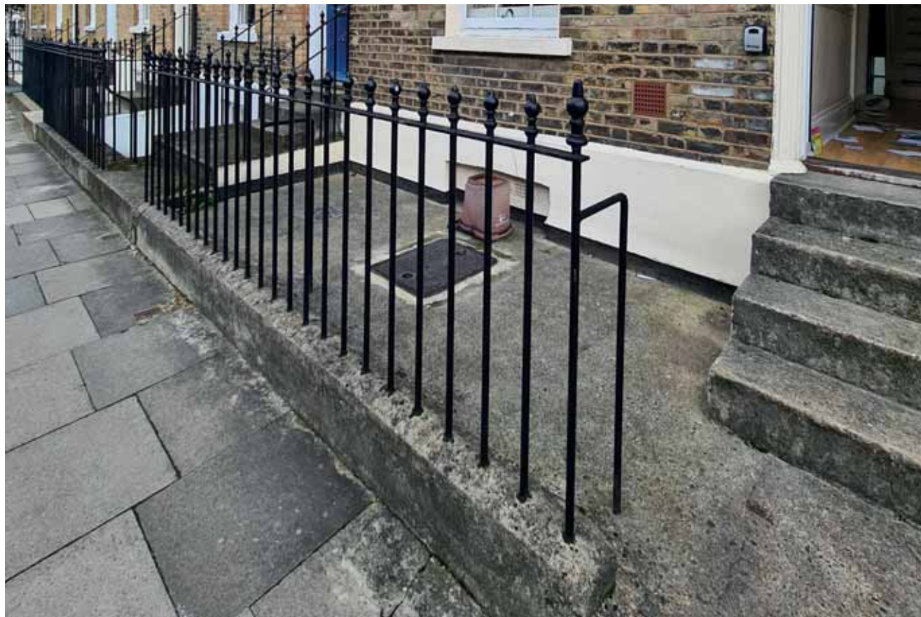
Existing front courtyard at No24
