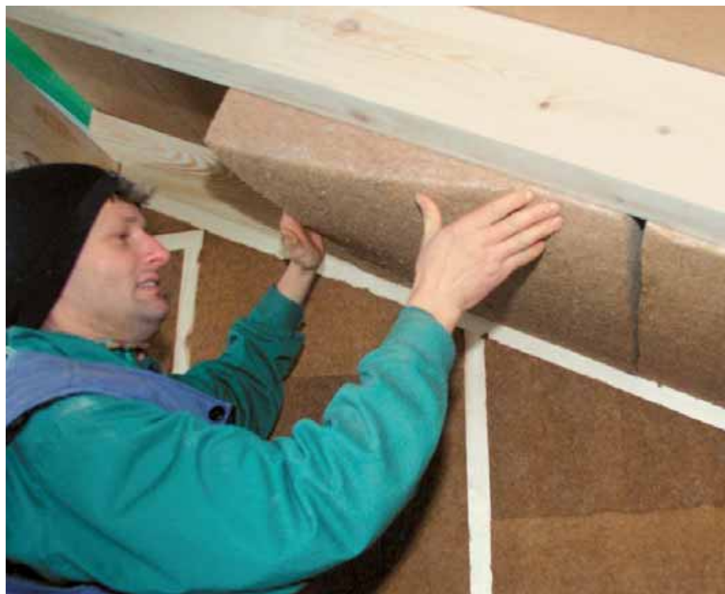
Example solution for internally upgrading the energy performance of roofs with natural insulation.
