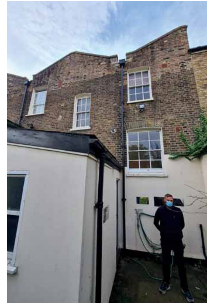
Existing Rear Elevation/Extension
