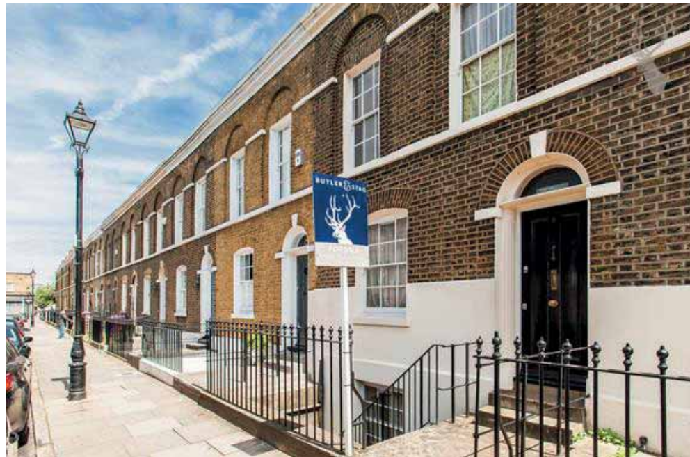
Railings and staircase to lower ground of No6 Aberavon Road
