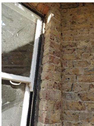
Figure 6: Straight brick joint exposed
