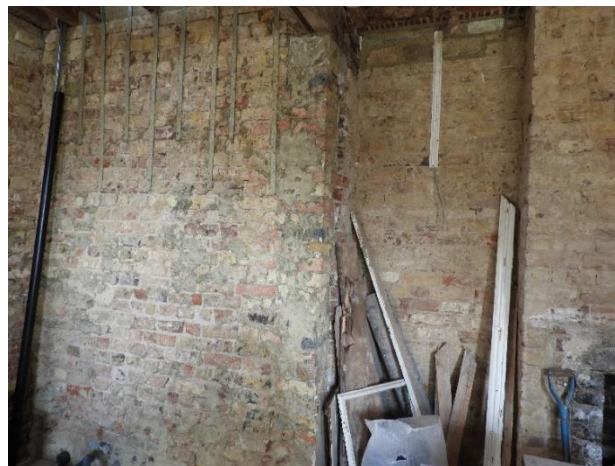
Figure 8: Interior wall of single storey extension to dwelling, butt jointed to original exterior wall
