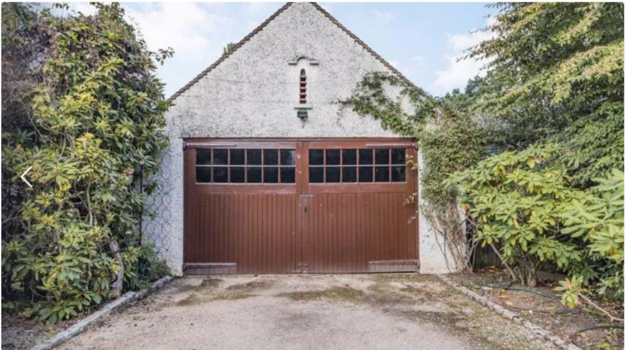
9. Front of garage/outbuilding
