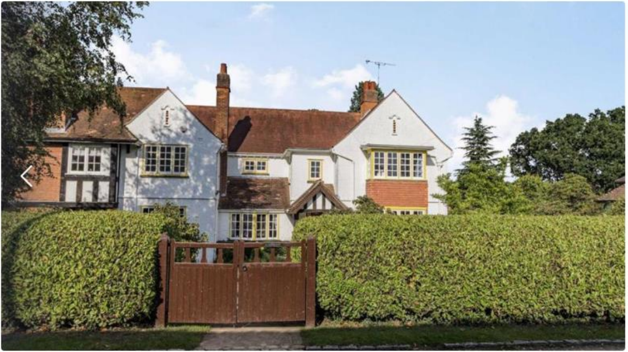
7a. Frontage of house
