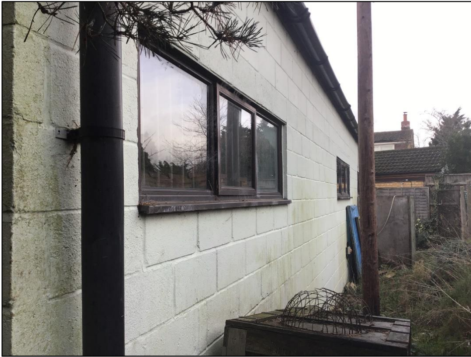
Plate 5: North aspect of building
