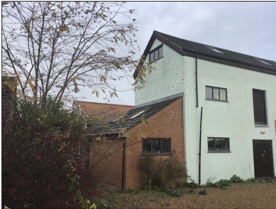
Plate 6: West aspect of building
