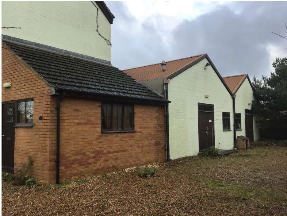
Plate 4: East aspect of building
