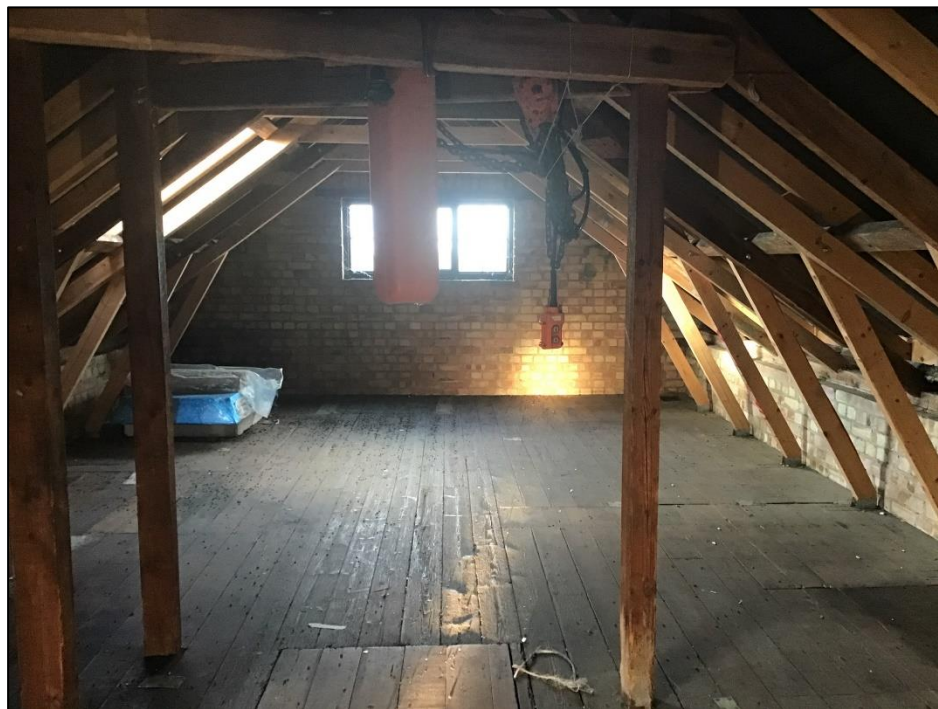
Plate 8: Interior of roof void to south
