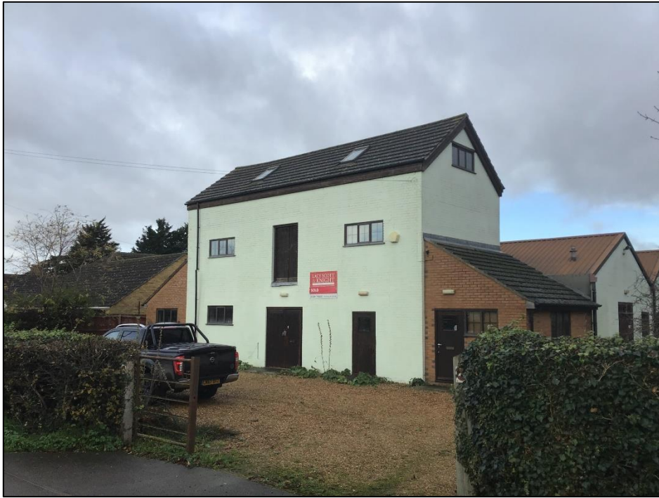
Plate 1: The site, showing north and east aspects of building
