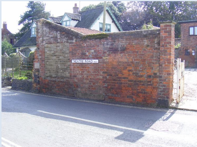
Section of wall inside conservation area
