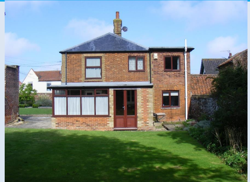
Rear of existing building
