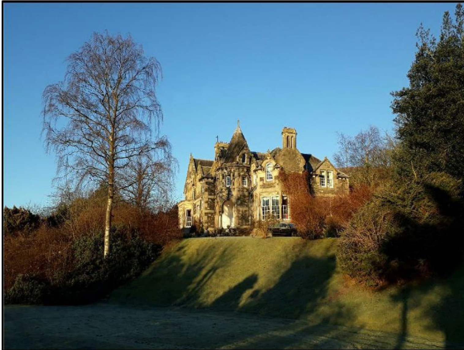
Photo 1 : The Kirna – Principal Elevations
