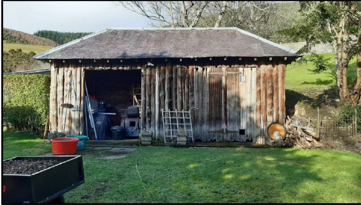
Photo 2 : South elevation of existing outbuilding to west of The Kirna.
