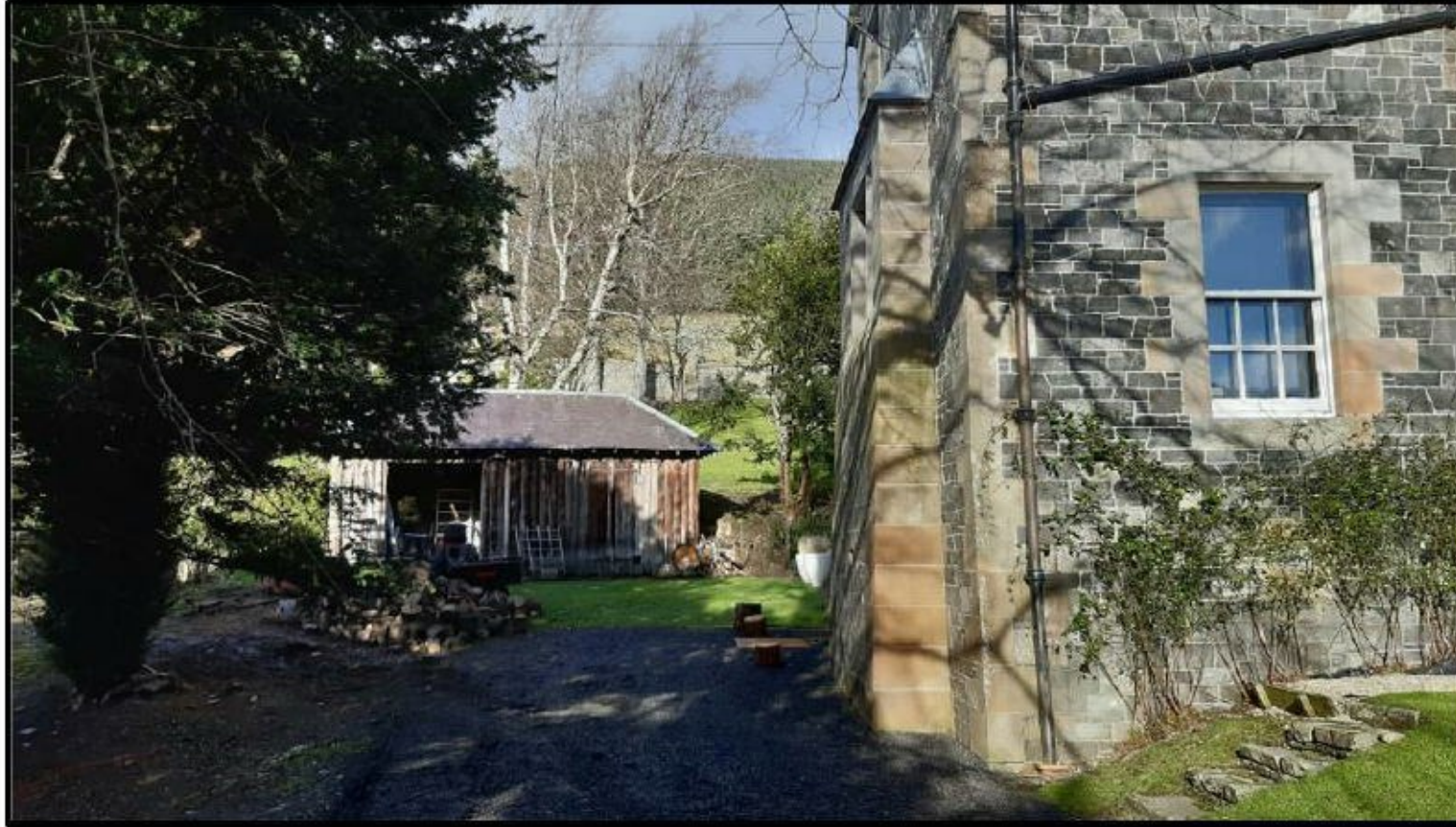
Photo 4 : South elevation of existing outbuilding to west of The Kirna in context.
