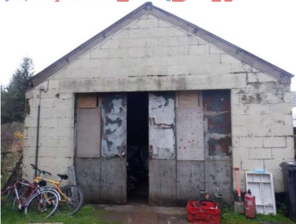
Figure 10 photo 9 view to south showing garage (L shaped building)
