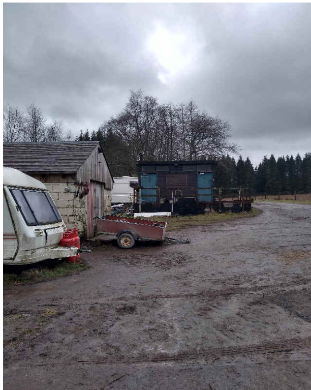
Existing Workshop & Public Conveniences – April 2022
