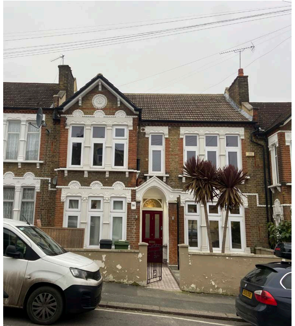
16 Shell Road | Front Elevation
