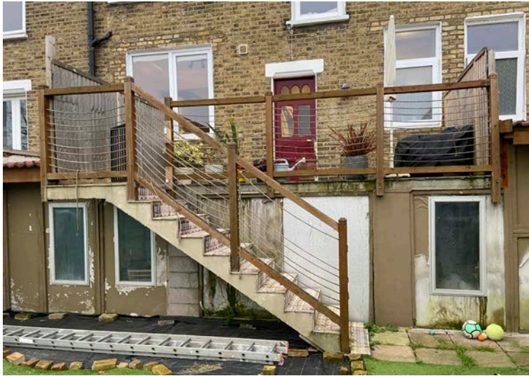
16 Shell Road | Rear Elevation
