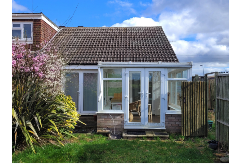
Existing Rear Elevation Site Photo
