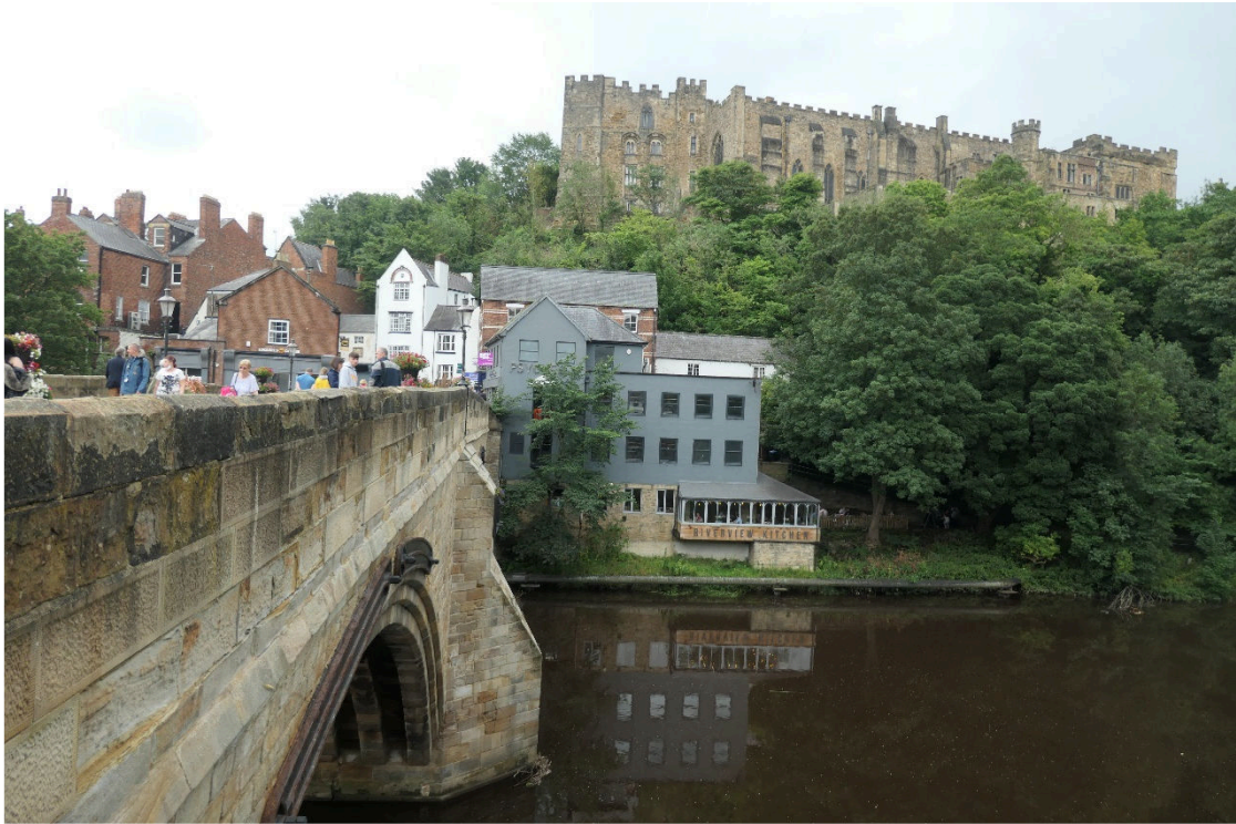
View from Framwellgate Bridge western abutment with the roof of No. 18 part visible
