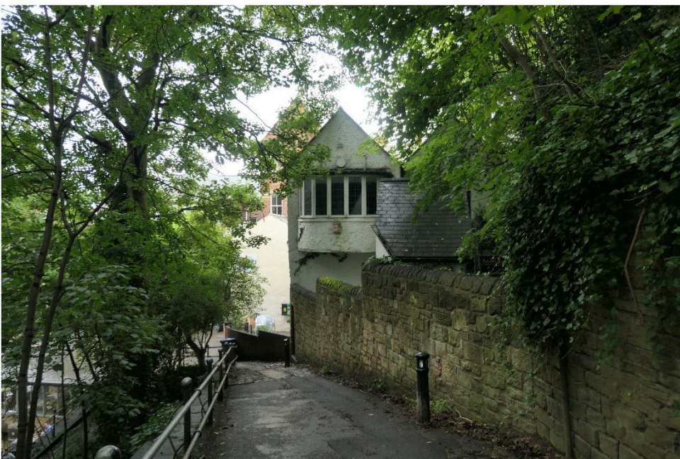
View from the public footpath to the rear of the site
