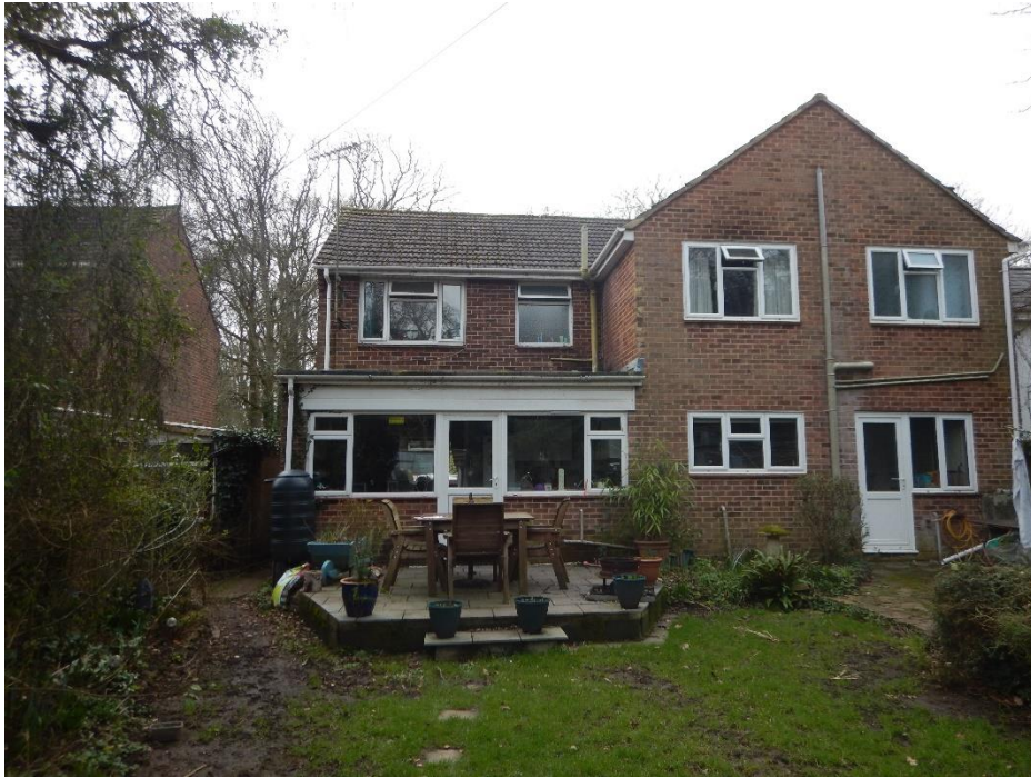
Existing rear of Treetops
